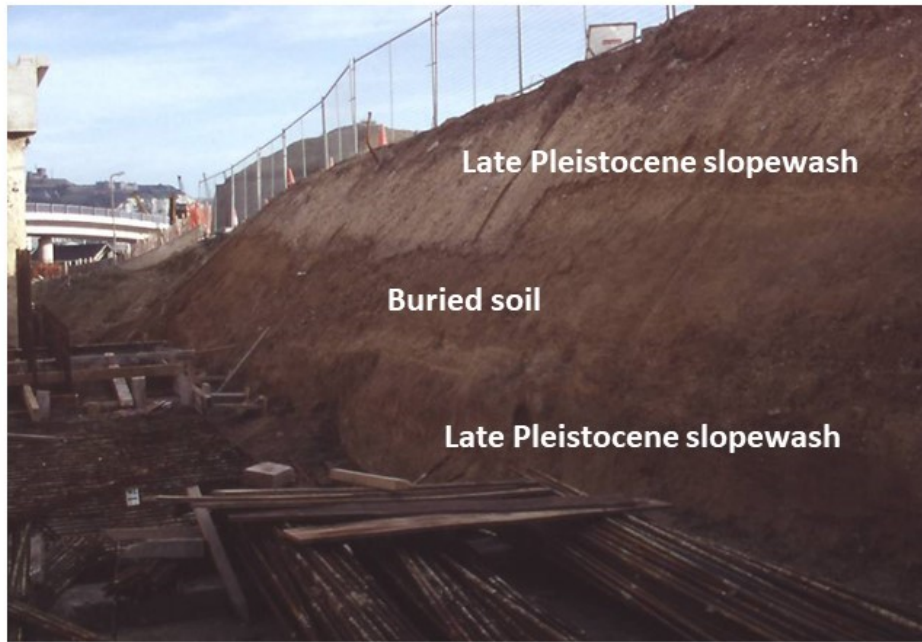
Figure 7. Slopewash and buried soils of Late Pleistocene age at Archcliffe Fort, Dover.
