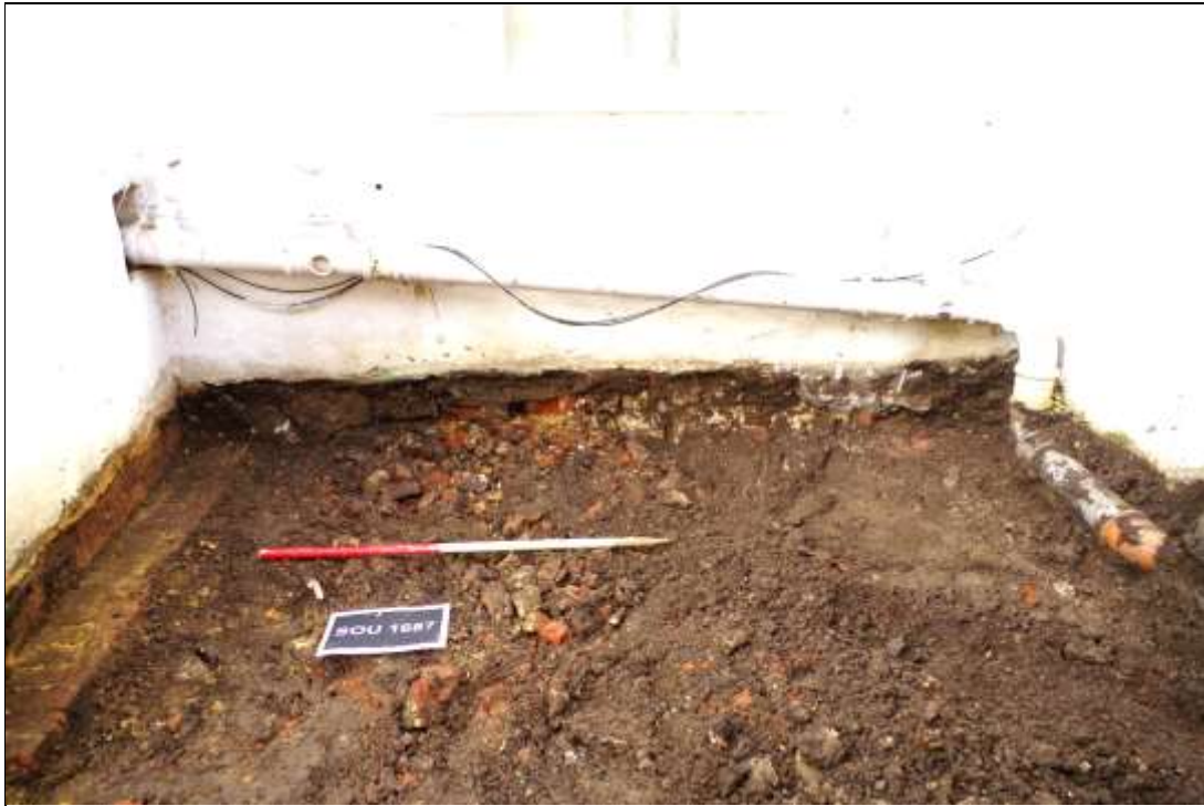
Figure 8. West corner of trench 1 showing layer 7, the brick and stone foundation 4 of Peartree House, and butress foundation 6 on the left.
