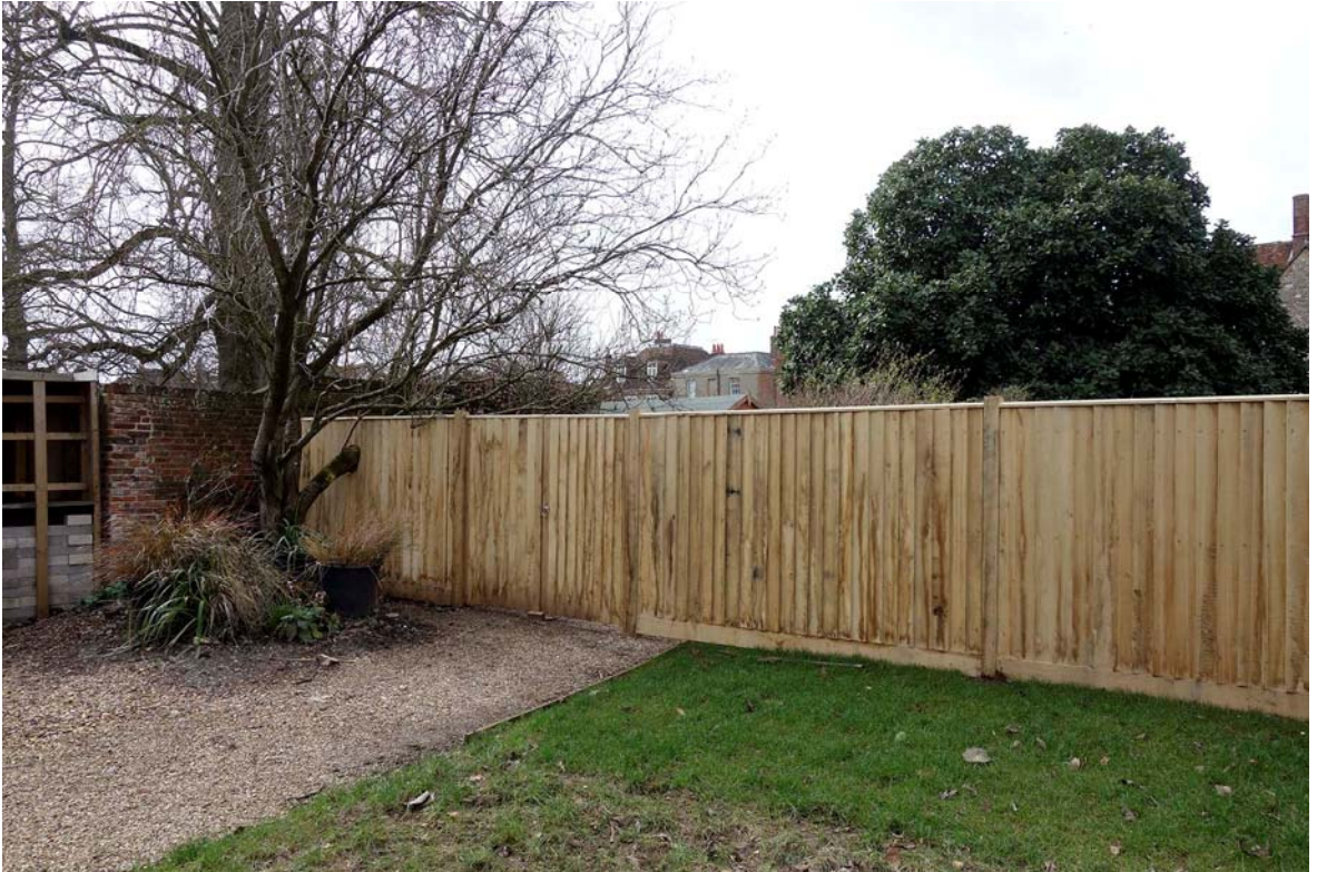
Figure 15. Fence completed, East side of bottom end.
