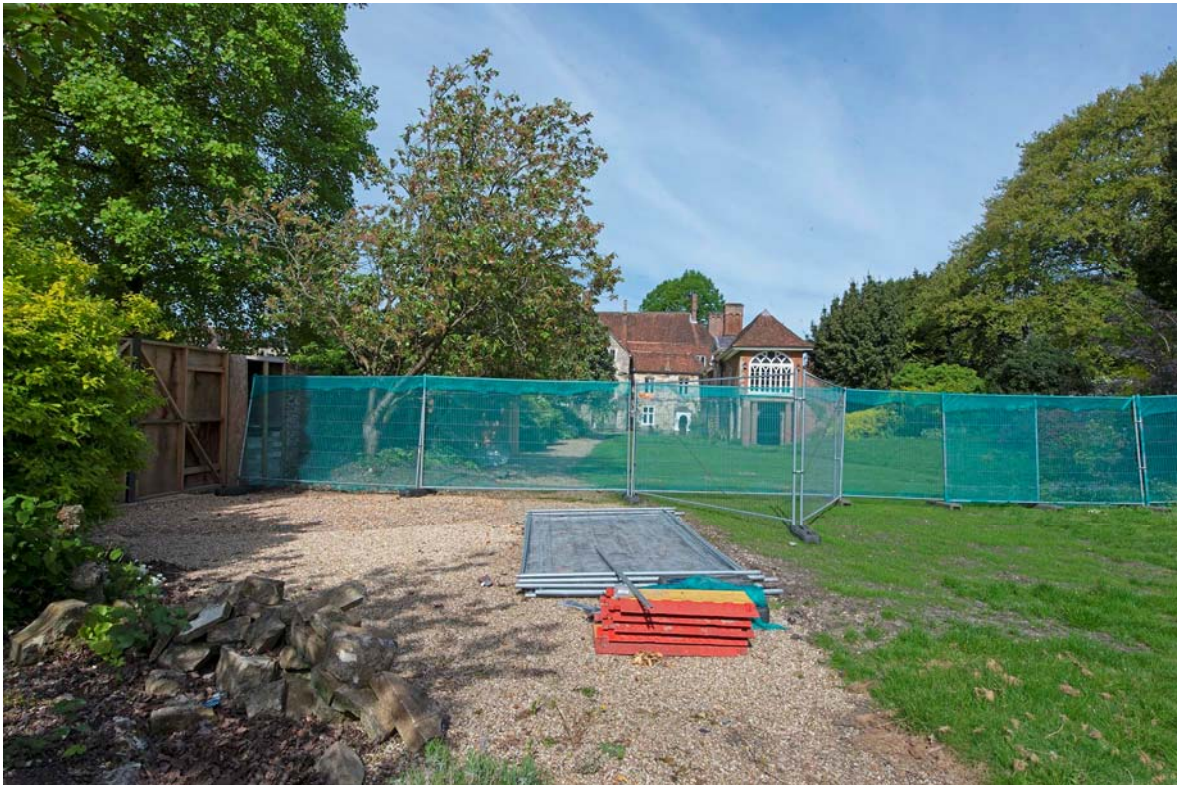
Figure 6. Pre-works view of south end of the site, looking west.
