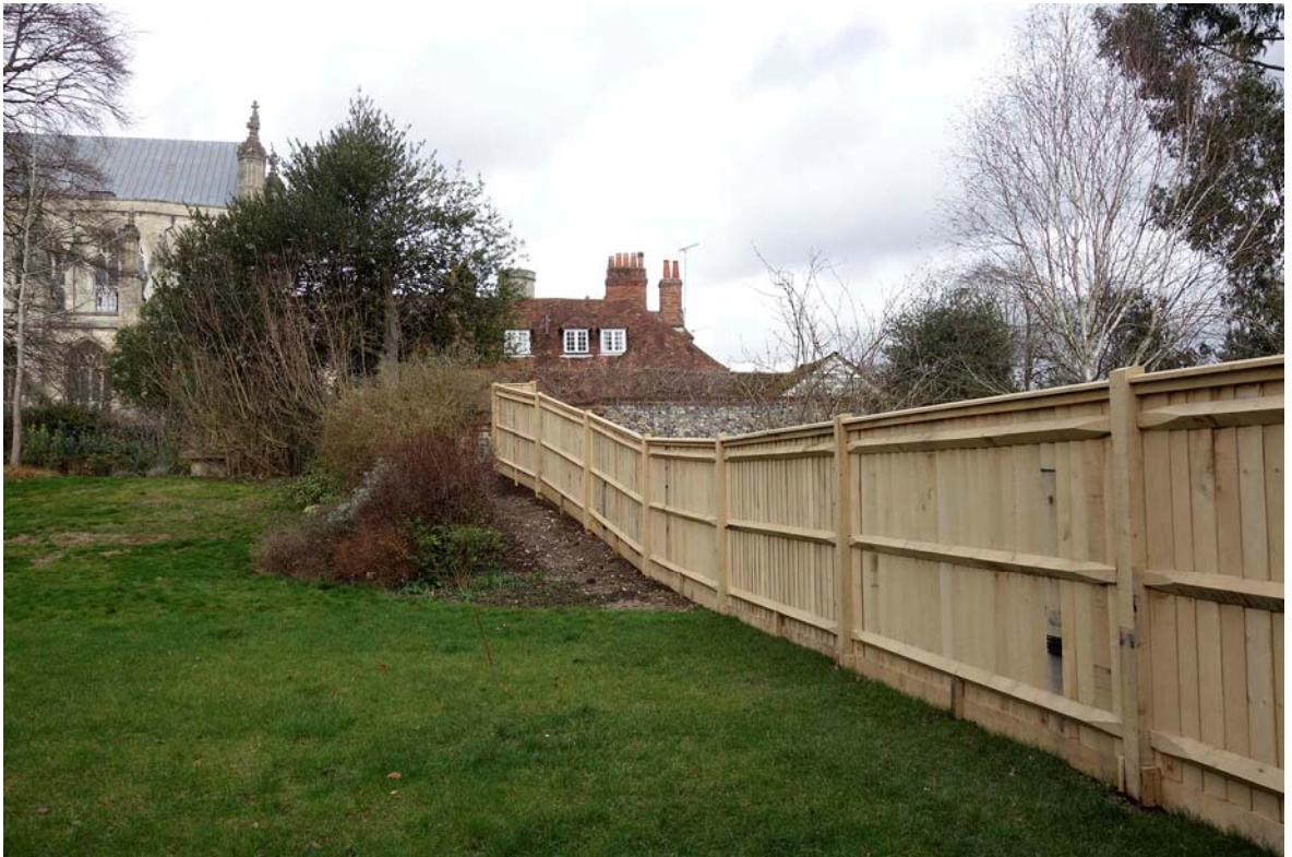
Figure 11. Fence completed, view NNE.
