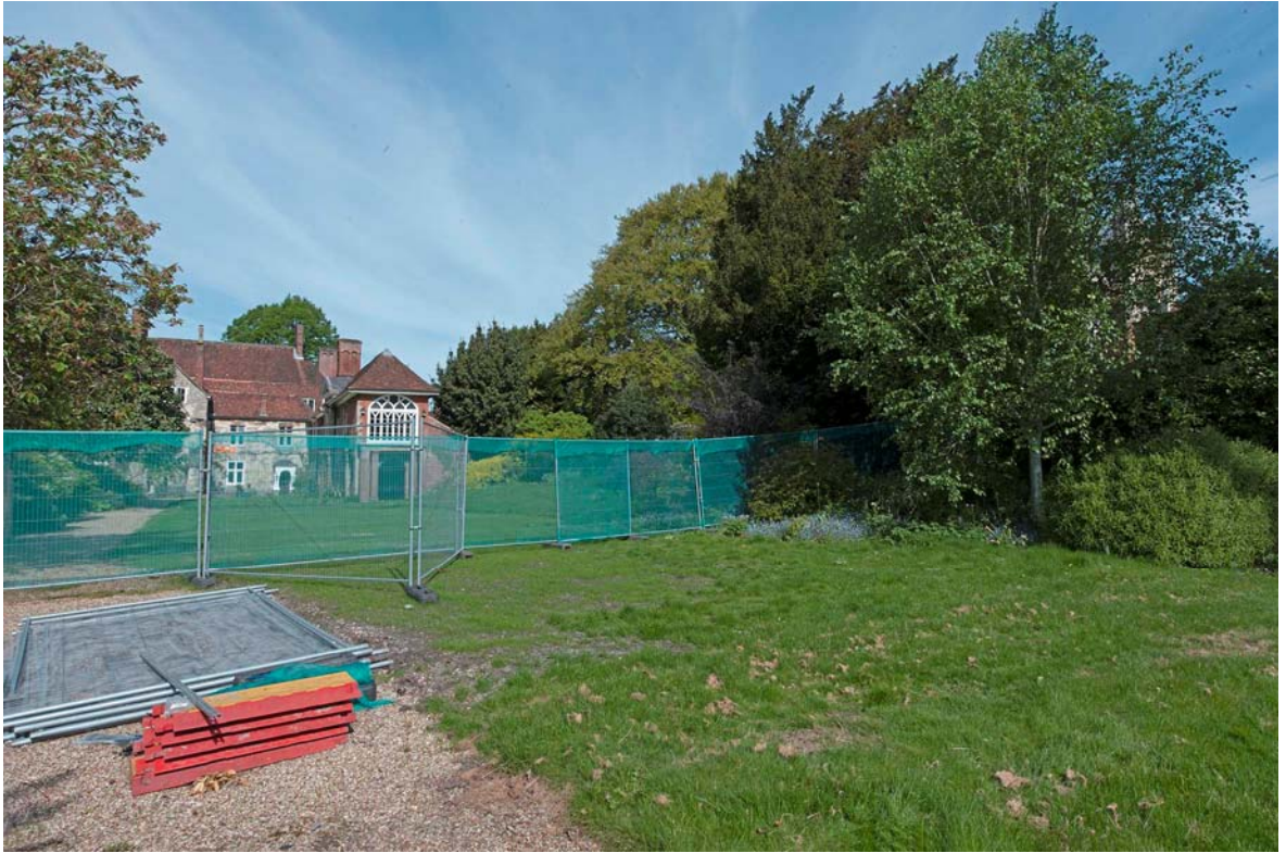
Figure 4. Pre-works view of the site, looking west.
