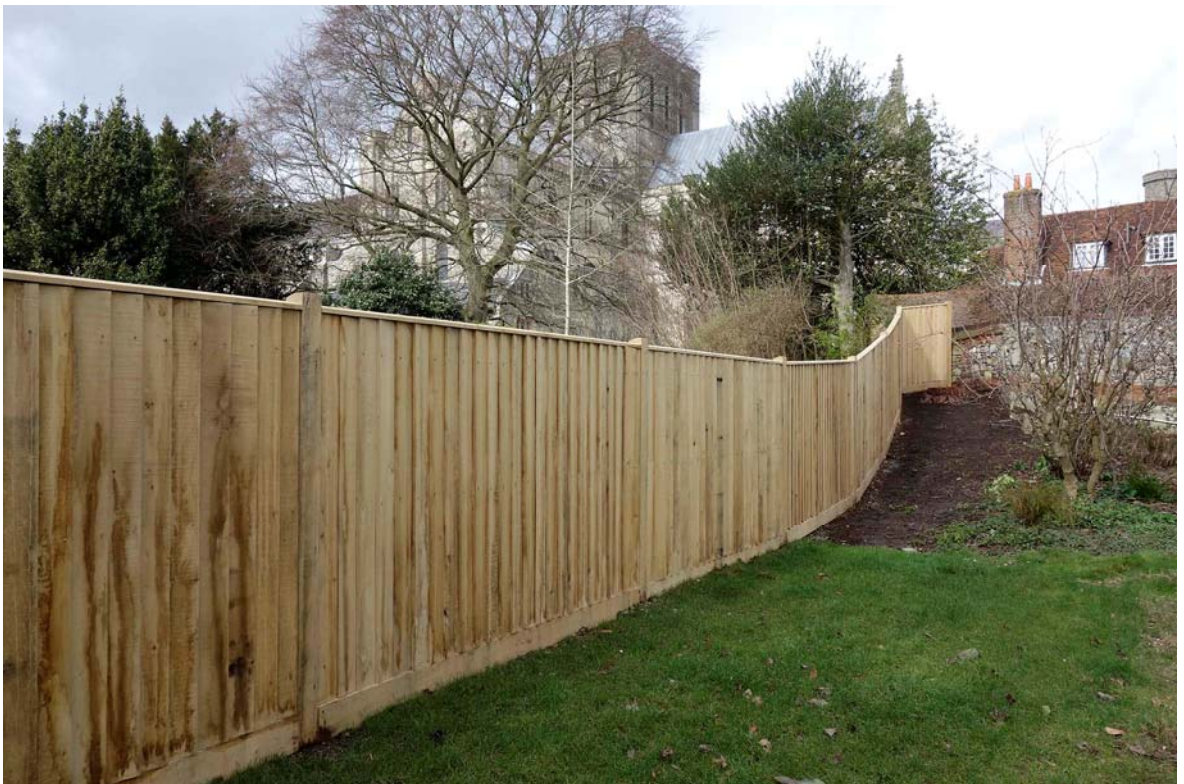
Figure 14. Fence completed. View NNW.
