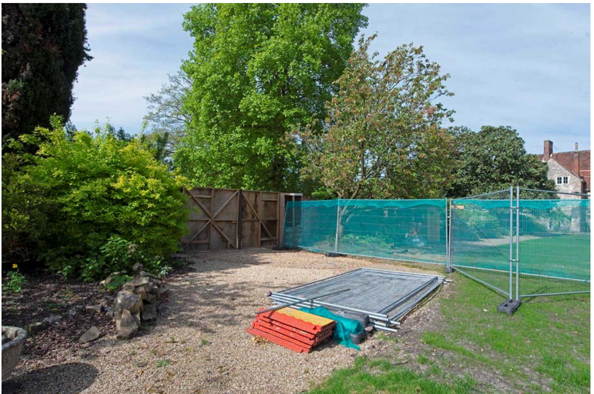
Figure 7. Pre-works view of the south end of the site looking south-west.
