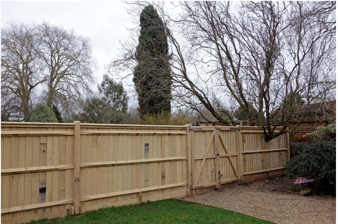
Figure 17. Fence completed. West side of south end.
