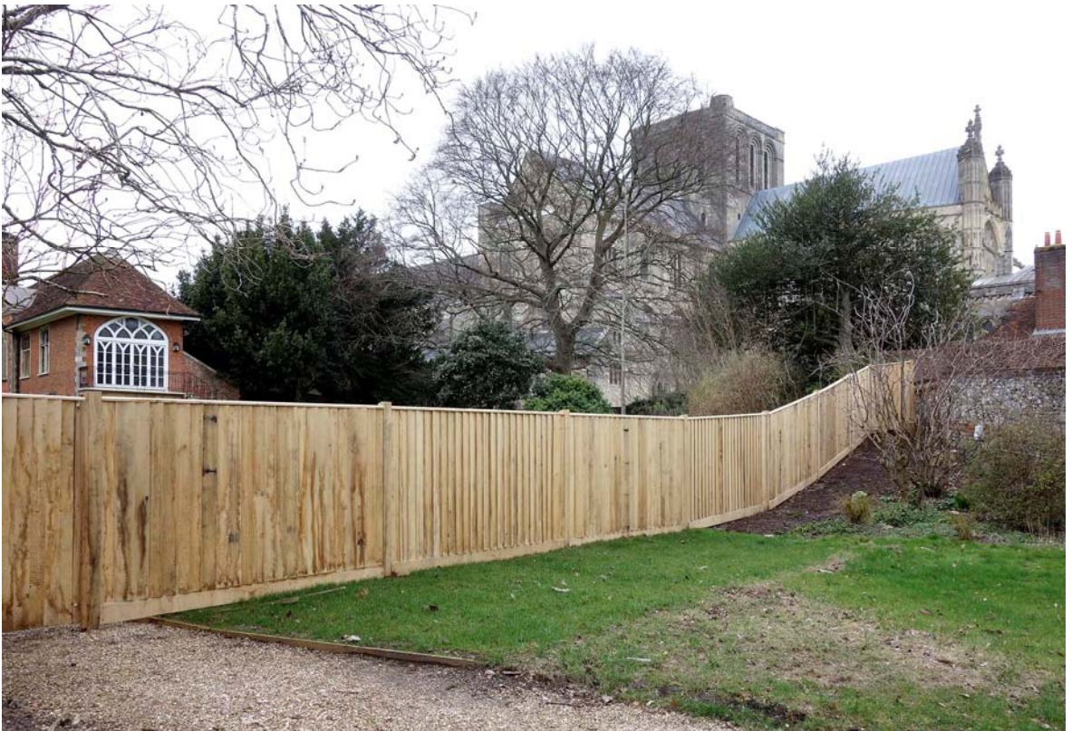
Figure 16. Fence completed. View north-west.
