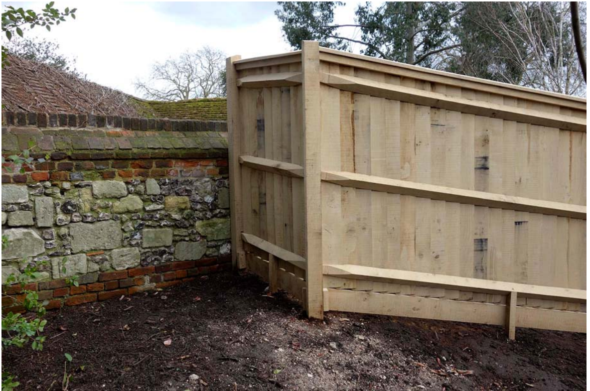
Figure 13. Fence completed. West side of top end.
