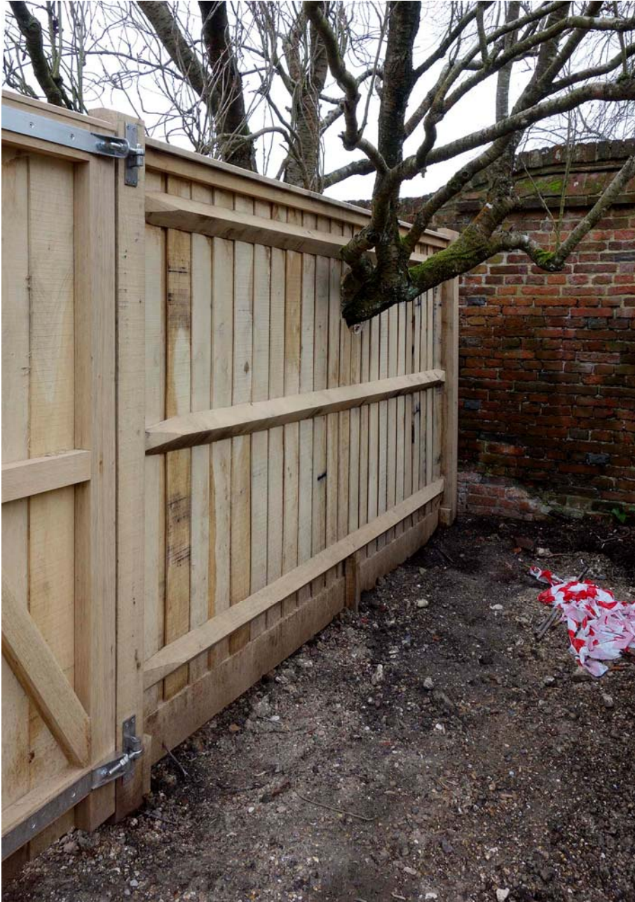
Figure 18. Fence completed. Accommodation of cherry tree.
