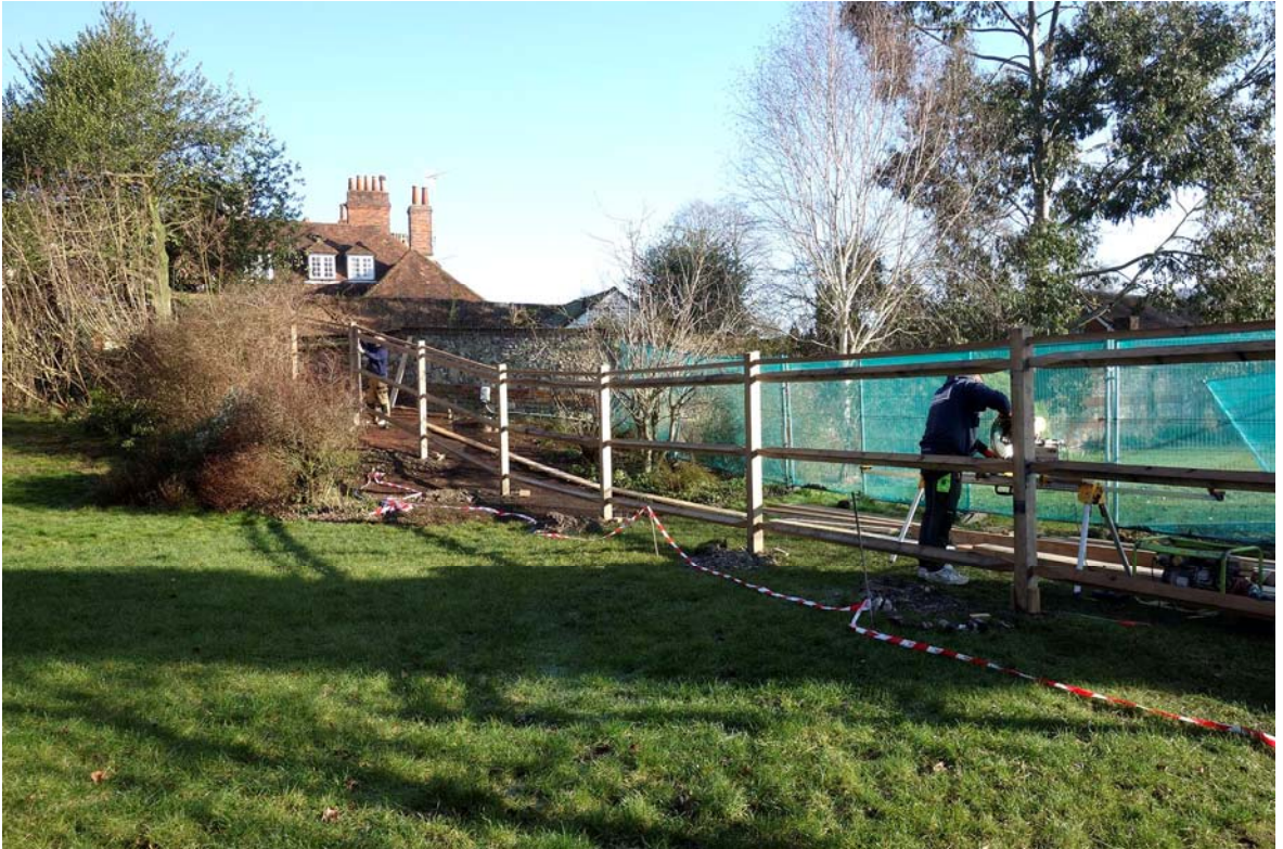
Figure 8. The fence under construction, looking NNE.
