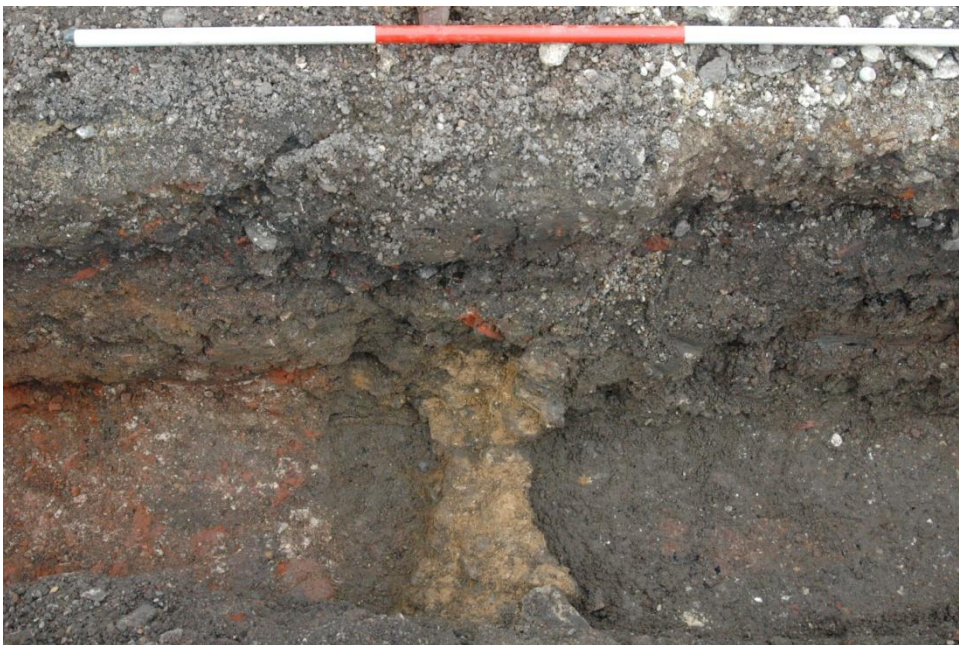
Plate 11: Wall plinth [0114], truncated by pits [0117] (left) and [0115] (right), and rubble filled trench [0121] (left), looking north.
