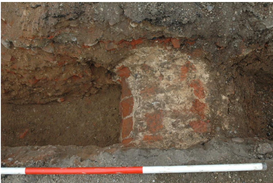
Plate 15: Demolished arch and abutment of bridge [0165] looking west, overlain by causeway infill to the south and abutted by gravel surfaces to the north
