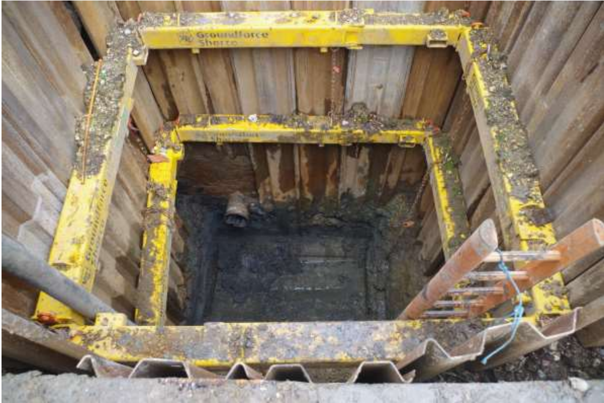
Plate 6. Natural deposits in base of northern manhole.
