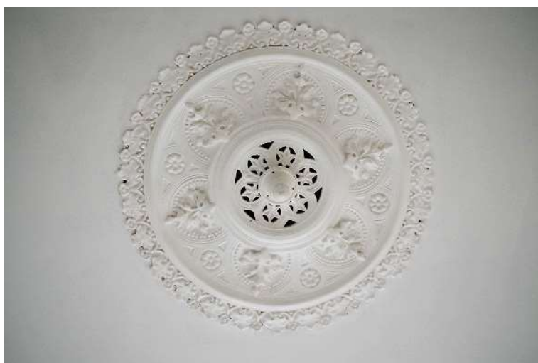
Moulding in centre of ceiling in Room 1
