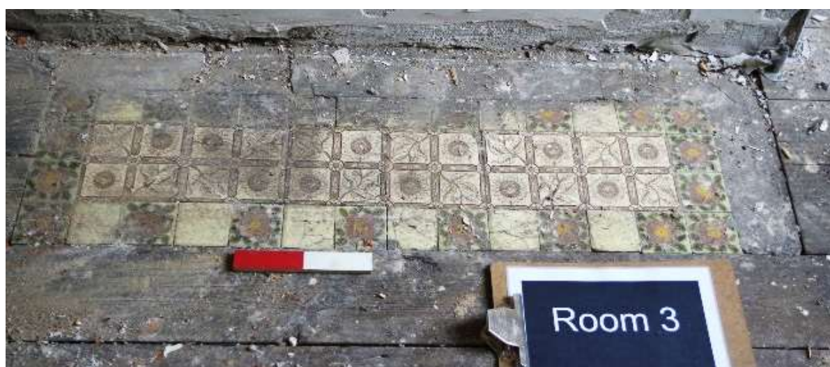
Tiles in front of chimney breast Room 3.
