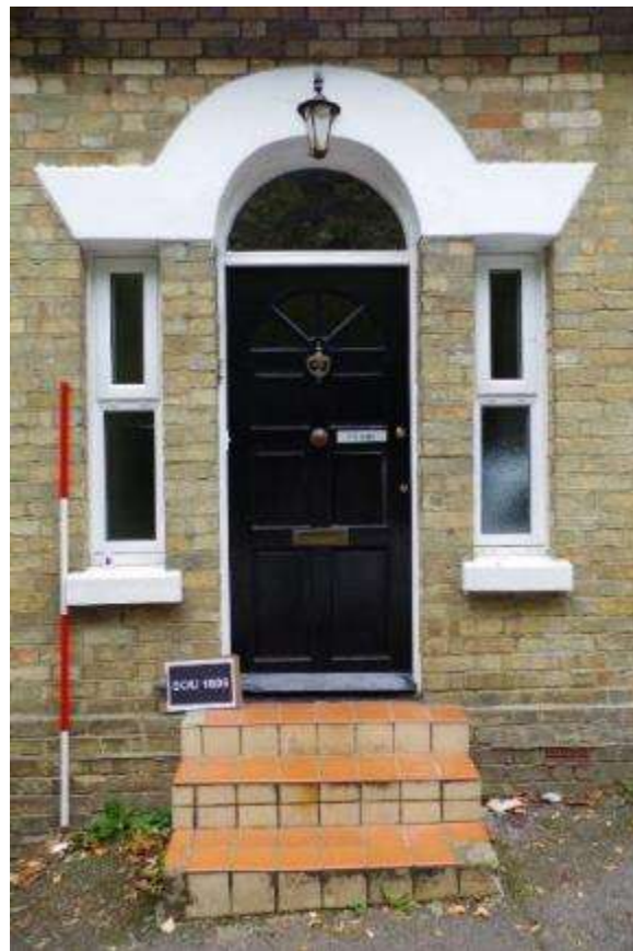
SW-facing elevation of external door and its venetian arch.
