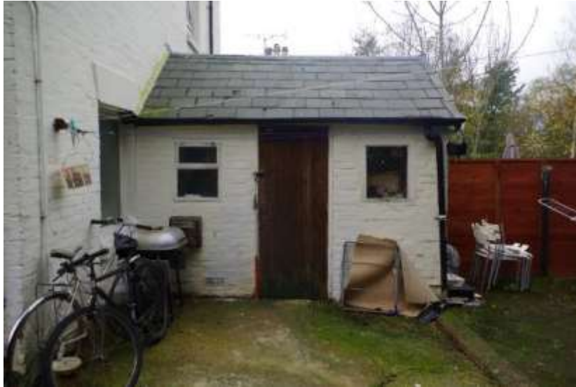
Northeast elevation of outhouse to 119, looking southwest
