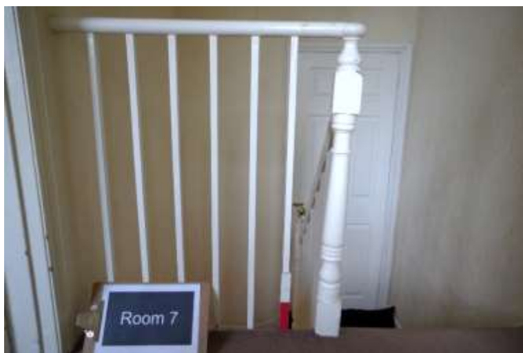
SW-facing elevation of 1 st Floor banister Room 7.
