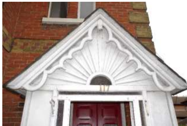
Close-up of SE-facing elevation of porch
