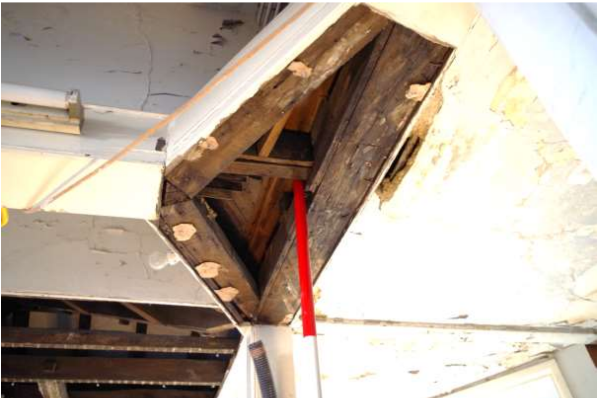
Figure 15. The Y-shaped arrangement of timbers supporting the lead pipe.
