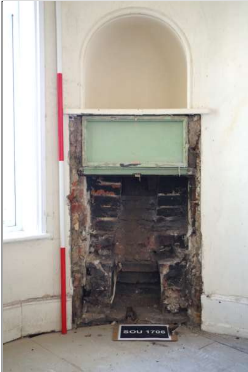
Figure 17. The fireplace in Flat 6 first floor.
