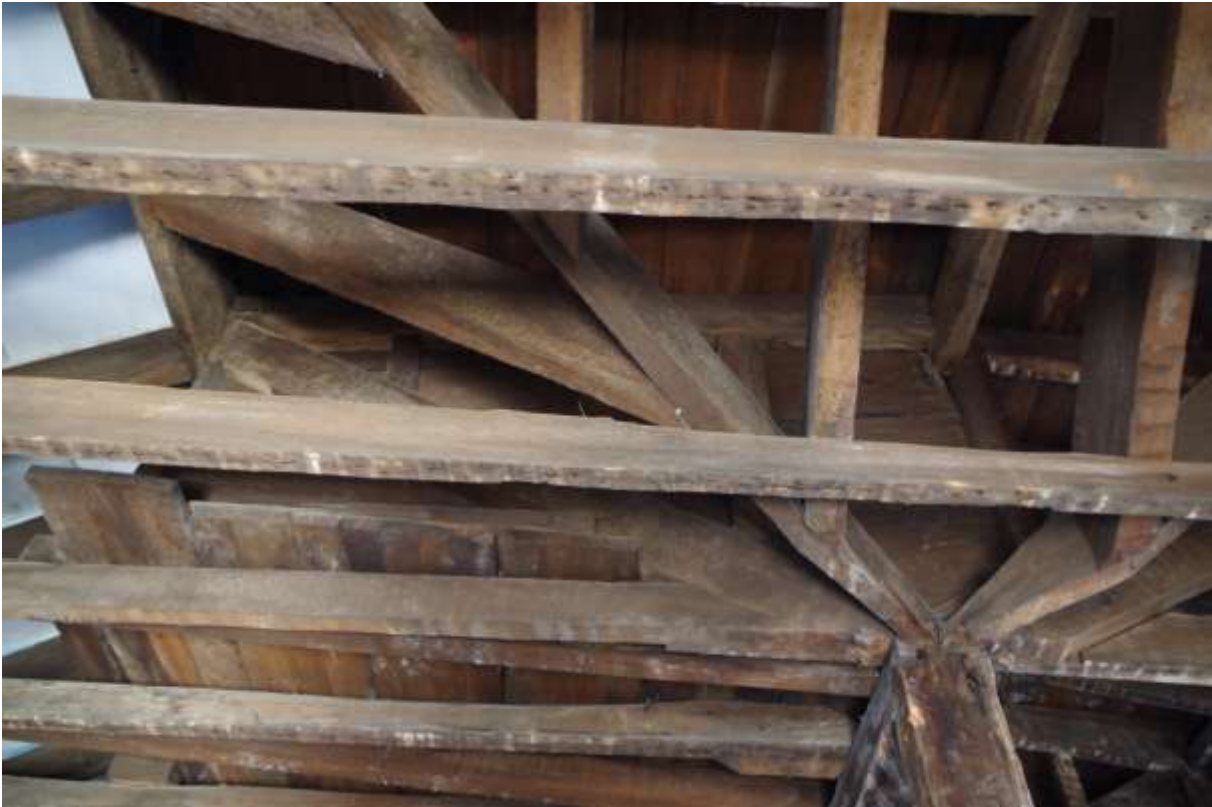
Figure 12. The attic roof structure after removal of ceilings. The original flat roof/light well structure formed from softwood planks can be seen above the joists.
