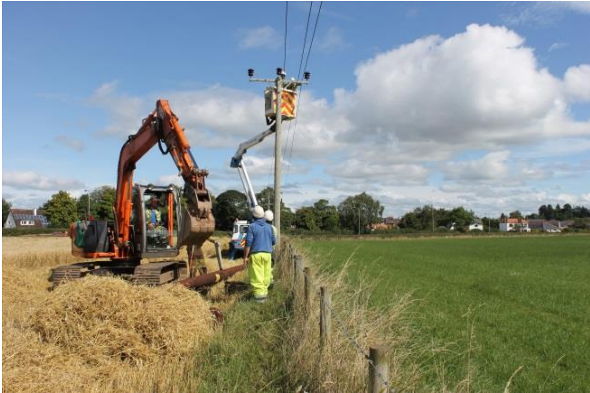
Fig. 7 Pole 1082542 – view from south
