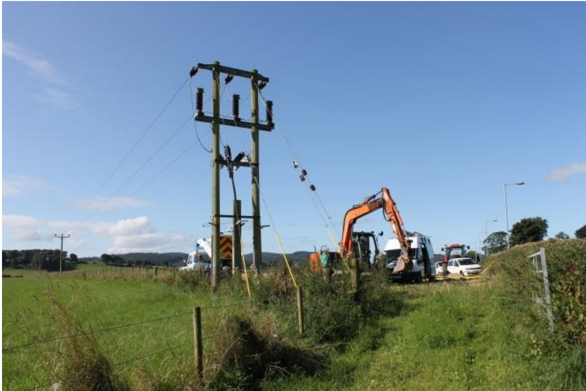
Fig.5. Pole 10792267 – view from east
