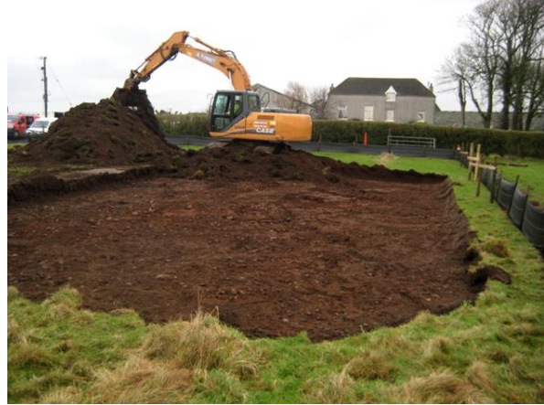
Fig 3. Site during machine excavation.
