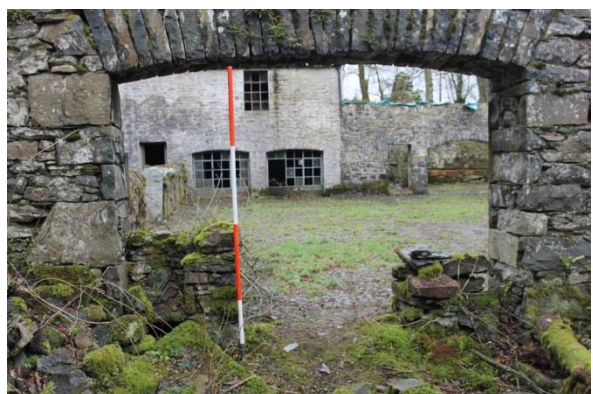
Fig 15. Building 1b entrance with blocking walls.
