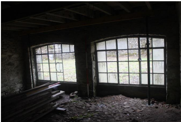
Fig 37. Building 5a interior.
