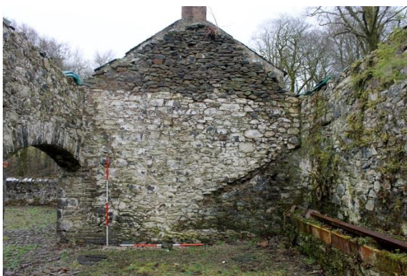
Fig 32. Building 4a, lean-to roof line + troughs.
