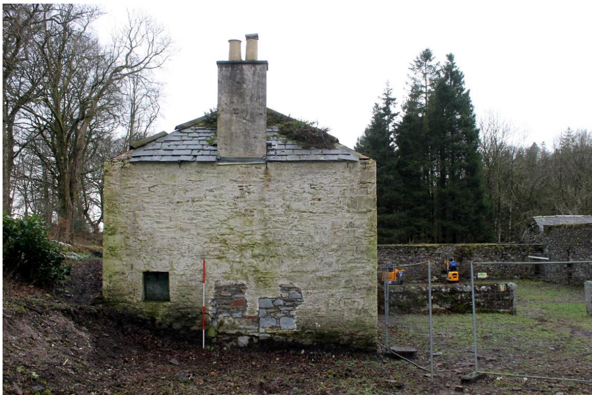
Fig 35. Building 5, NE end with hipped roof.
