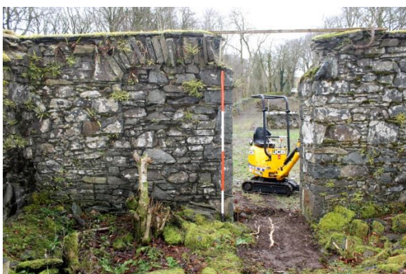
Fig 26. Building 3b door and arch (?) stones.
