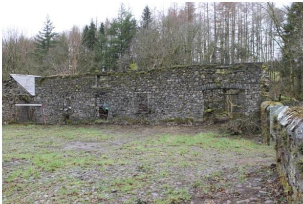
Fig 16. Buildings 1 b and c from SE.
