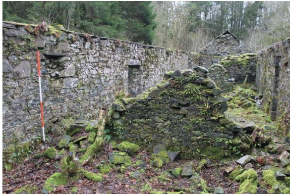
Fig 28. Building 3d, view to NW.
