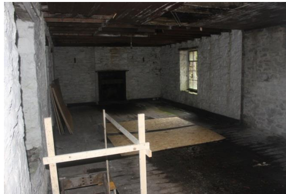
Fig 38. Building 5d interior, view SE.
