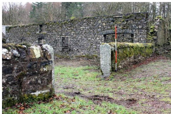
Fig 40. Dividing wall of courtyards and Building 1
