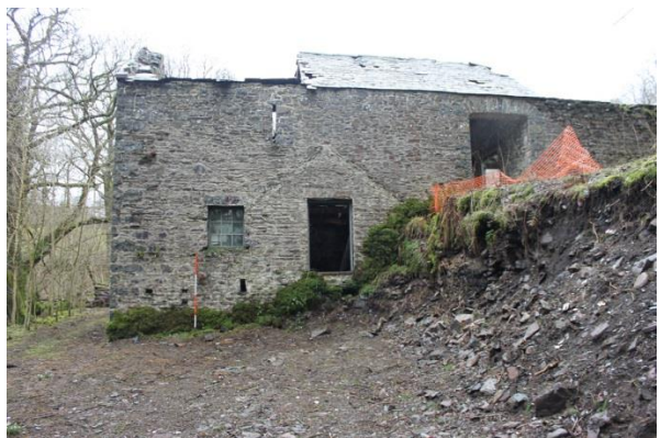
Fig 21. Building 2 from SW.
