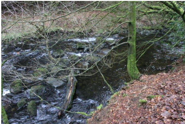
Fig 10 Stone weir and lade take-off channel.
