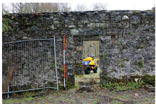
Fig 27. Building 3c doorways from SW.
