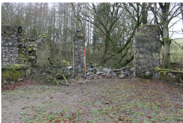
Fig 14. Building 1a from SE.
