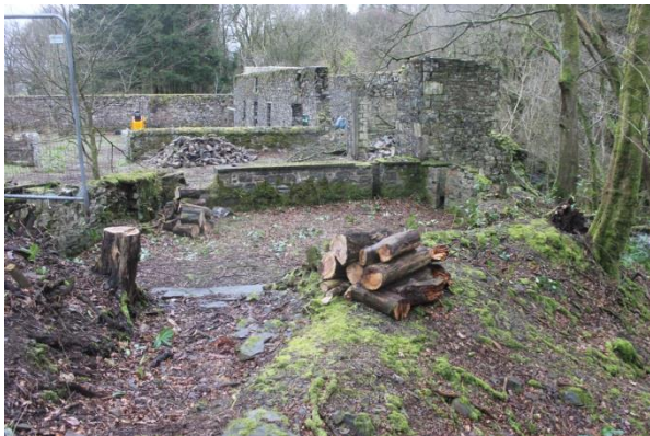
Fig 12. Holding pond from NE.
