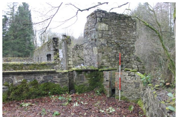
Fig 13. Overflow (right) and culvert recess (centre).
