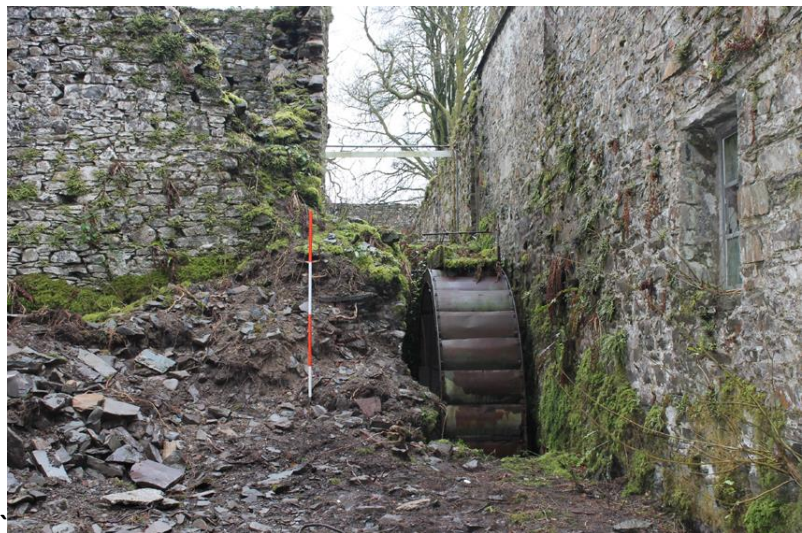
Fig 19. Mill wheel from NW, Building 2b to right.
