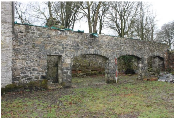
Fig 30. Building 4a from NW.
