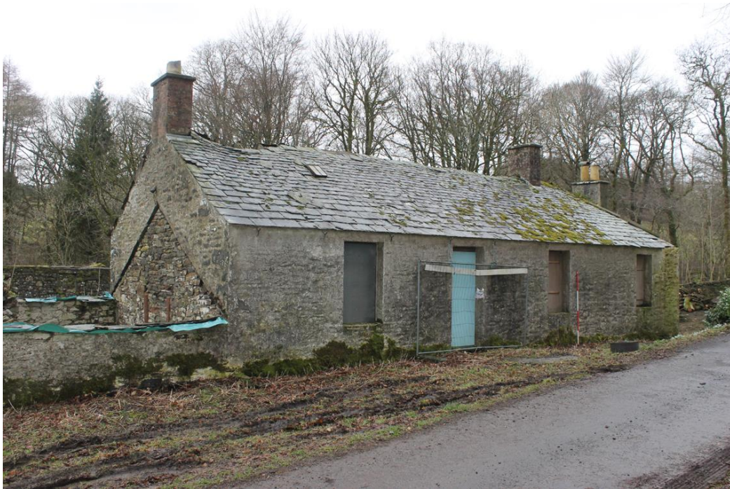
Fig 36. Building 5, view of cottage from road.
