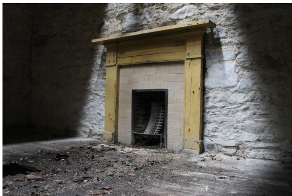
Fig 39. Building 5d, fireplace at NW end.
