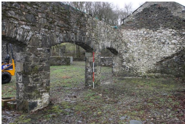
Fig 31. Building 4a interior.
