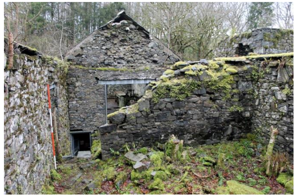
Fig 25. Buildings 3 a and b from SE.
