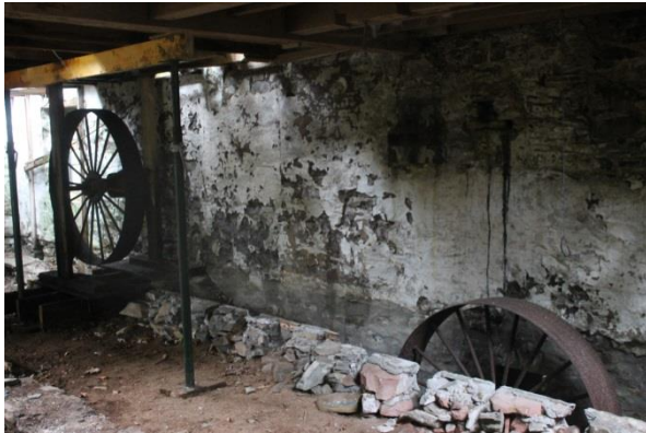
Fig 22. Building 2b pulley drives.
