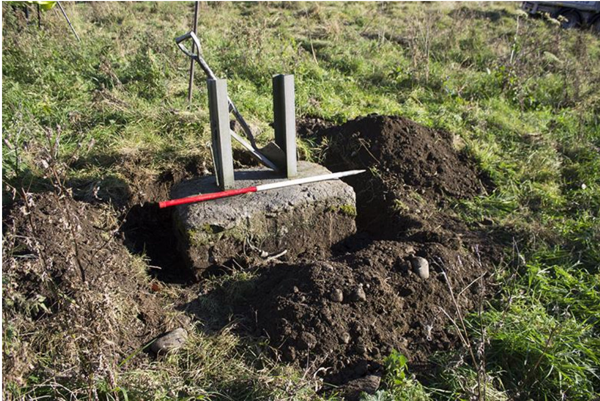
Fig 6. Base of Tower 1 after removal of tower structure.
