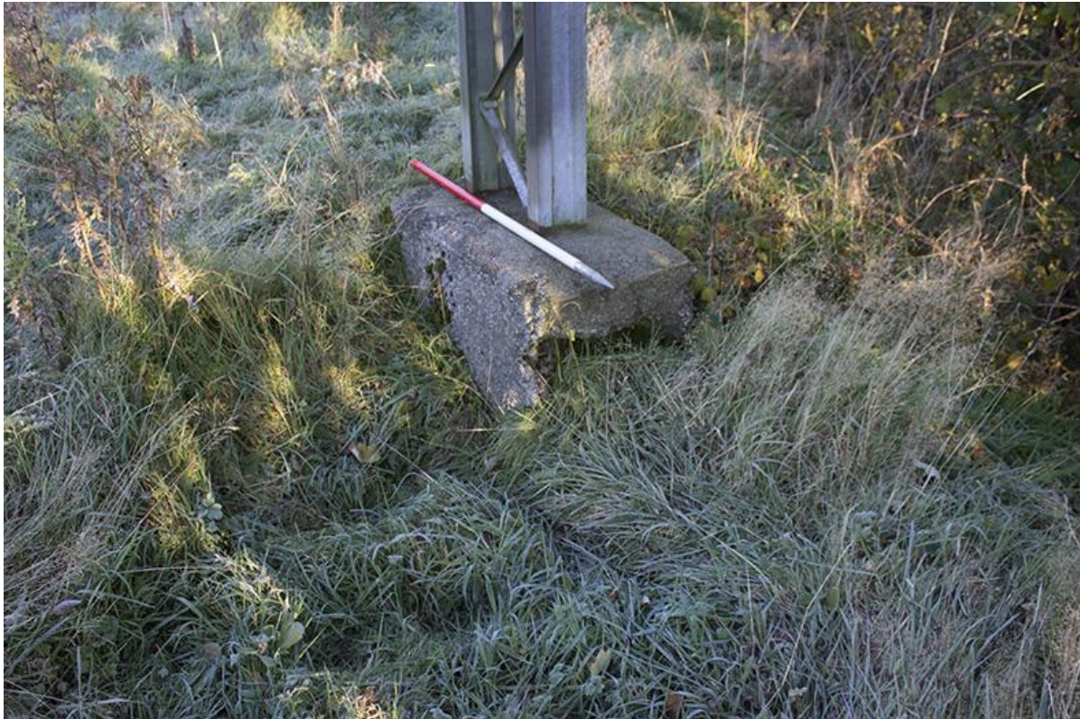
Fig 8. Tower 2, concrete base from south.
