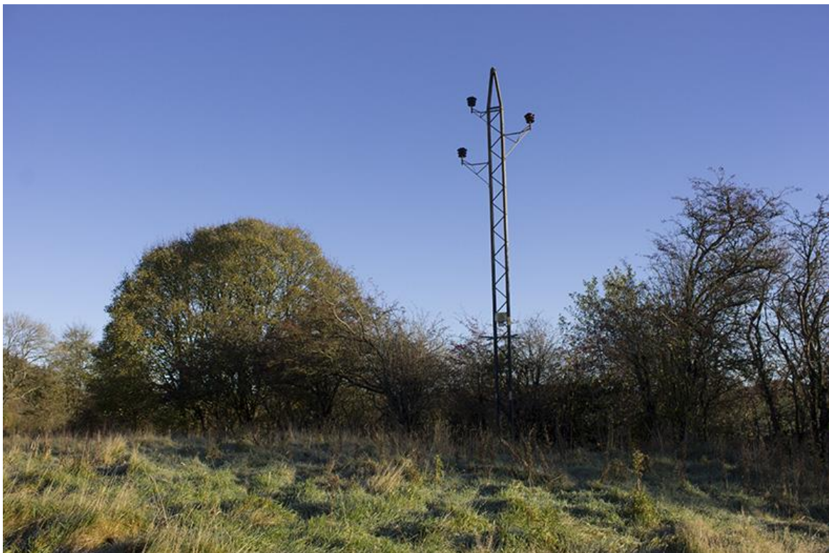
Fig 5. Tower 2 from south.
