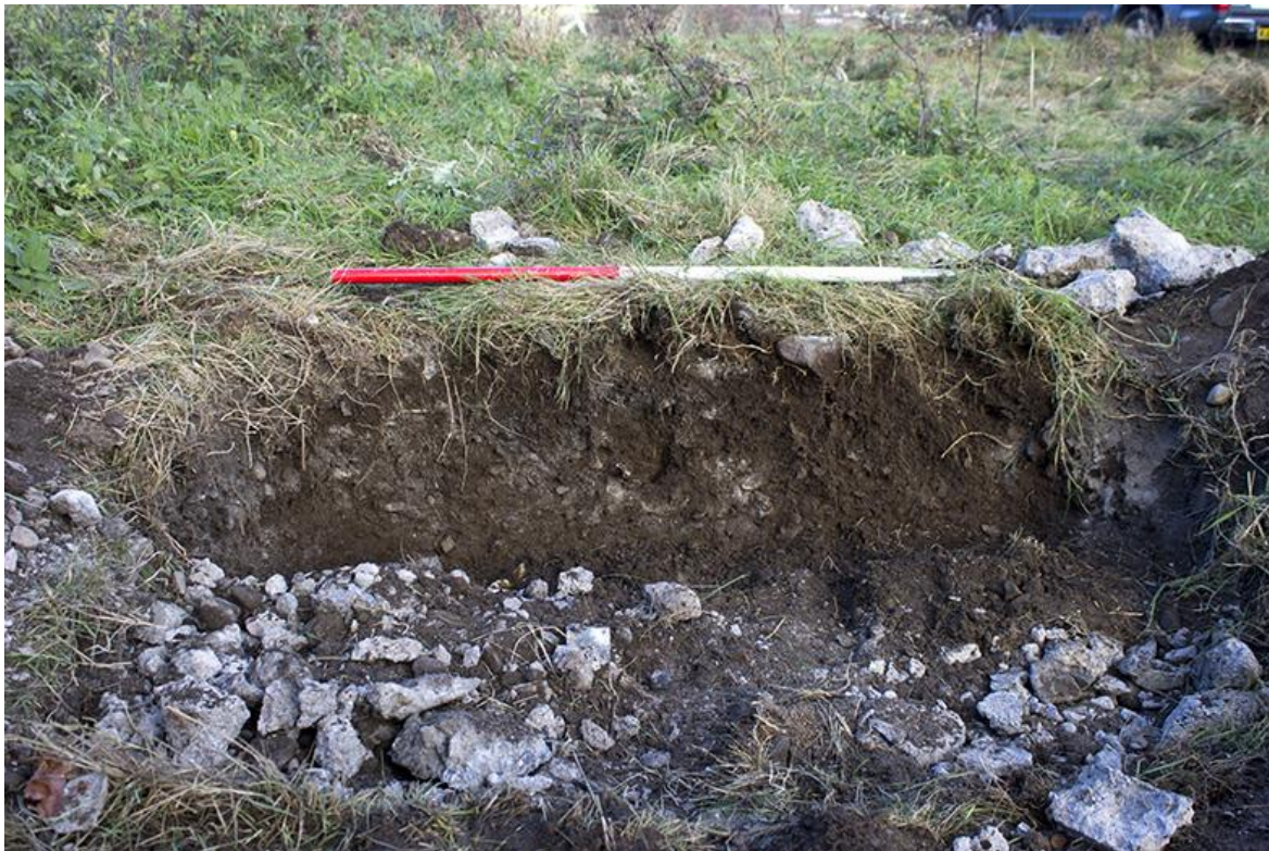
Fig 7. Tower 1, west facing elevation after reduction of concrete base.
