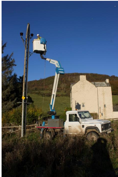
Fig 4. Tower 1 during removal of insulators.
