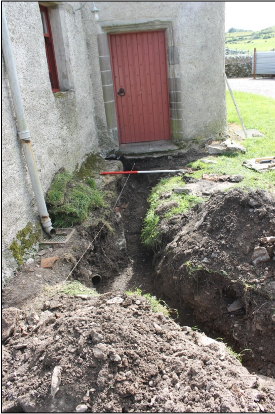
Fig. 9. Trench 1, general view.
