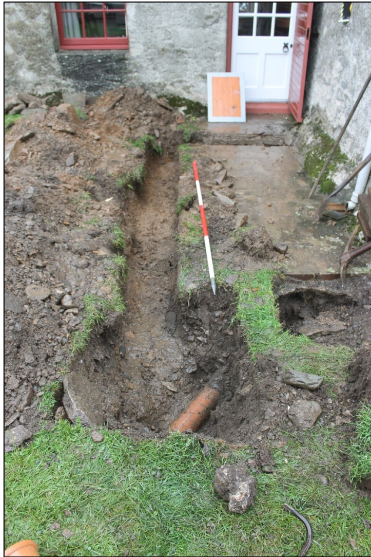
Fig.12. Trench 2. General post-excavation view with pipe (9) in foreground.
