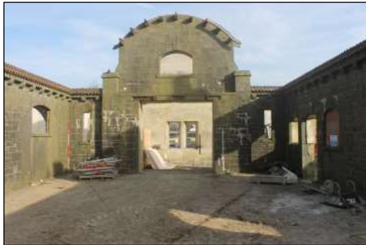
Plate 5. North Range barn, view north from courtyard
