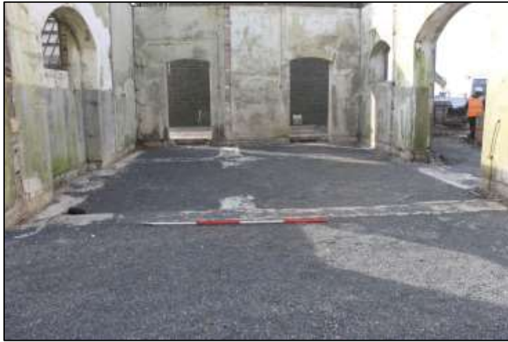
Plate 4. North Range cart shed interior, view south.
