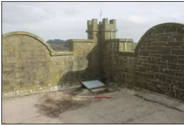
Plate 20. Tower yard showing crenellation and access to water tank.
