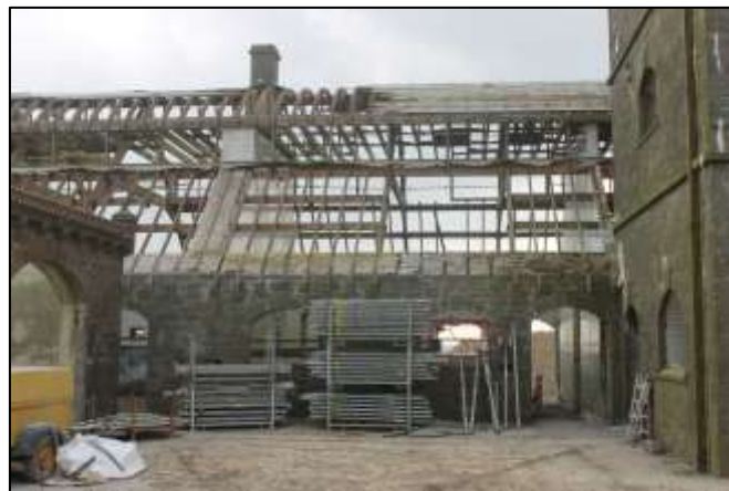
Plate 13. South Range north face viewed from courtyard.
