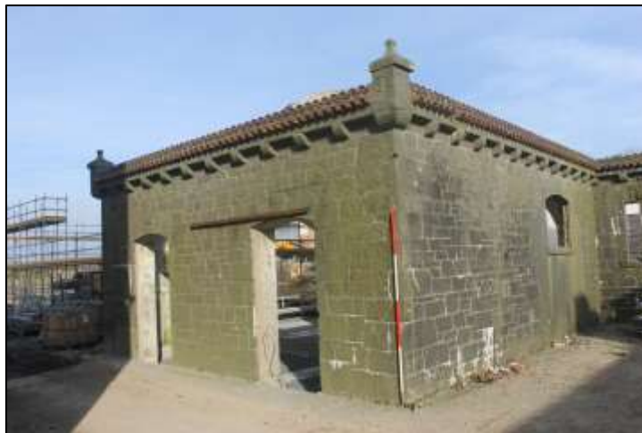
Plate 2. North Range cart shed from south-east..
