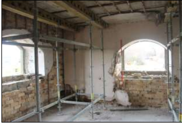
Plate 19. Tower second floor, view from south-west.
