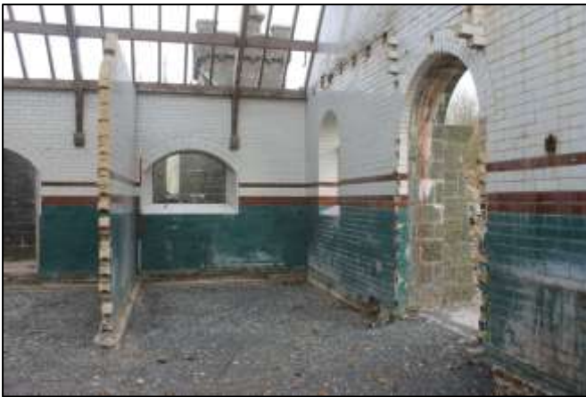
Plate 15. South Range (area 1), view from south-west.
