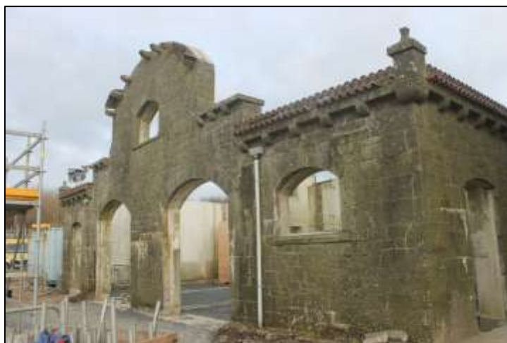
Plate 3. North Range cart shed, west face.
