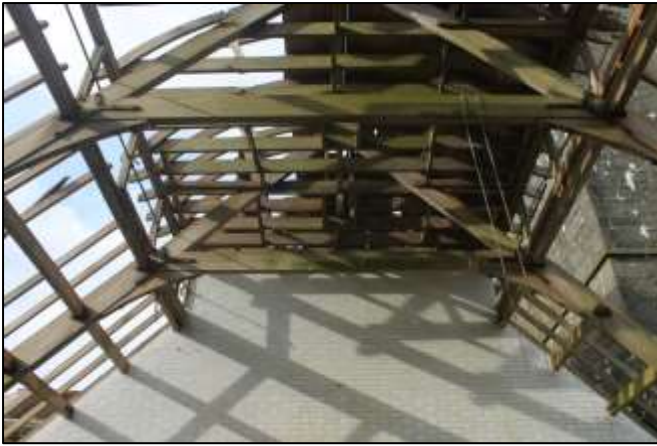
Plate 14. South Range roof.
