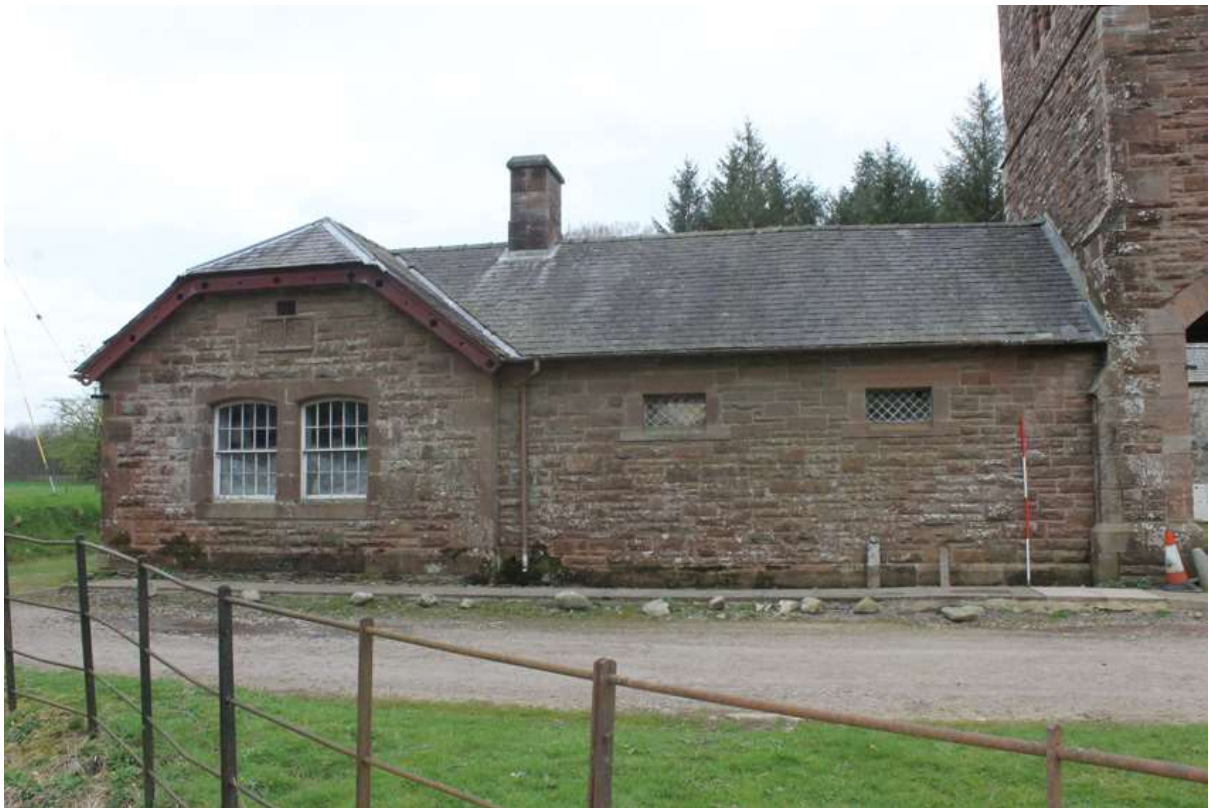
Fig. 19. East Wing – outer face of EW1 and 2.
