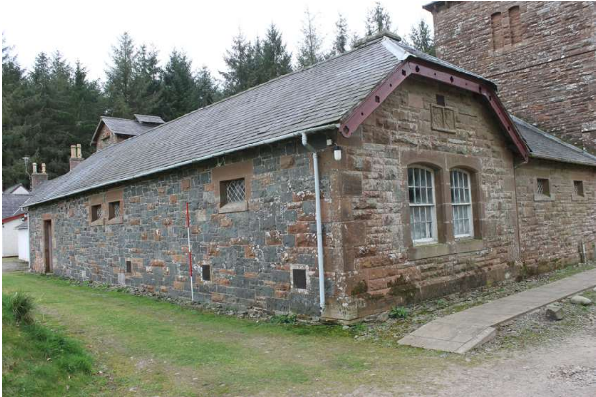
Fig. 14. South Wing – re-used armorial plaque above bipartite windows in SW4.
