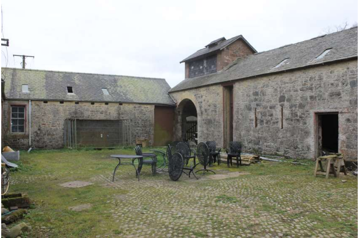
Fig. 8. West Wing – general view across courtyard with South Wing to left.
