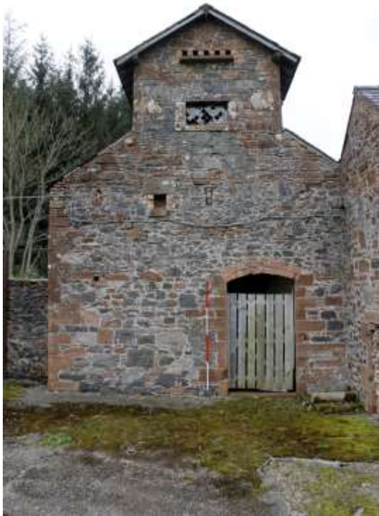
Fig. 12. West Wing – south gable with doocot and flight holes.
