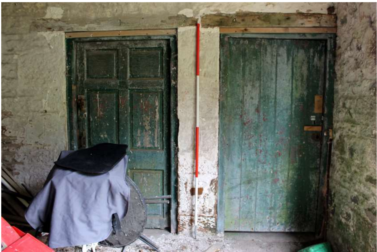
Fig. 17. South Wing – doors to SW3 and 4 from EW1.
