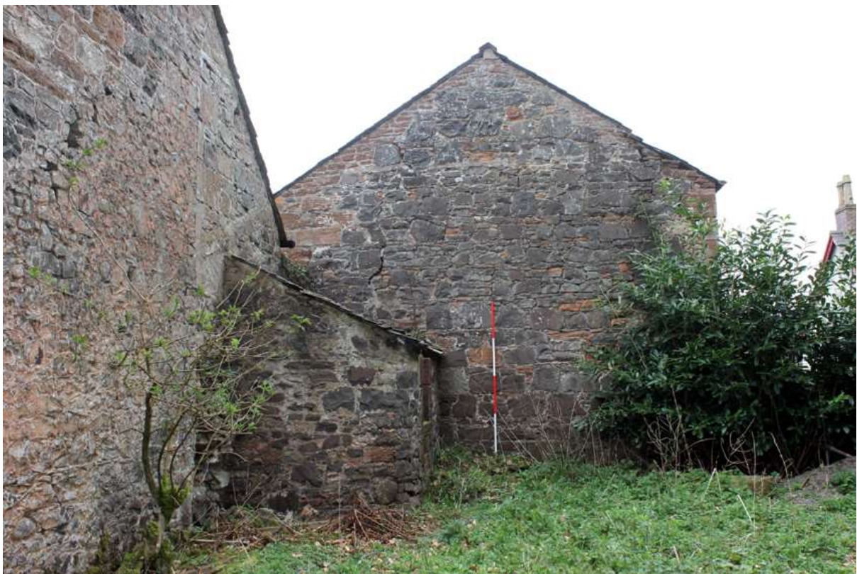
Fig. 11. West Wing – north gable.
