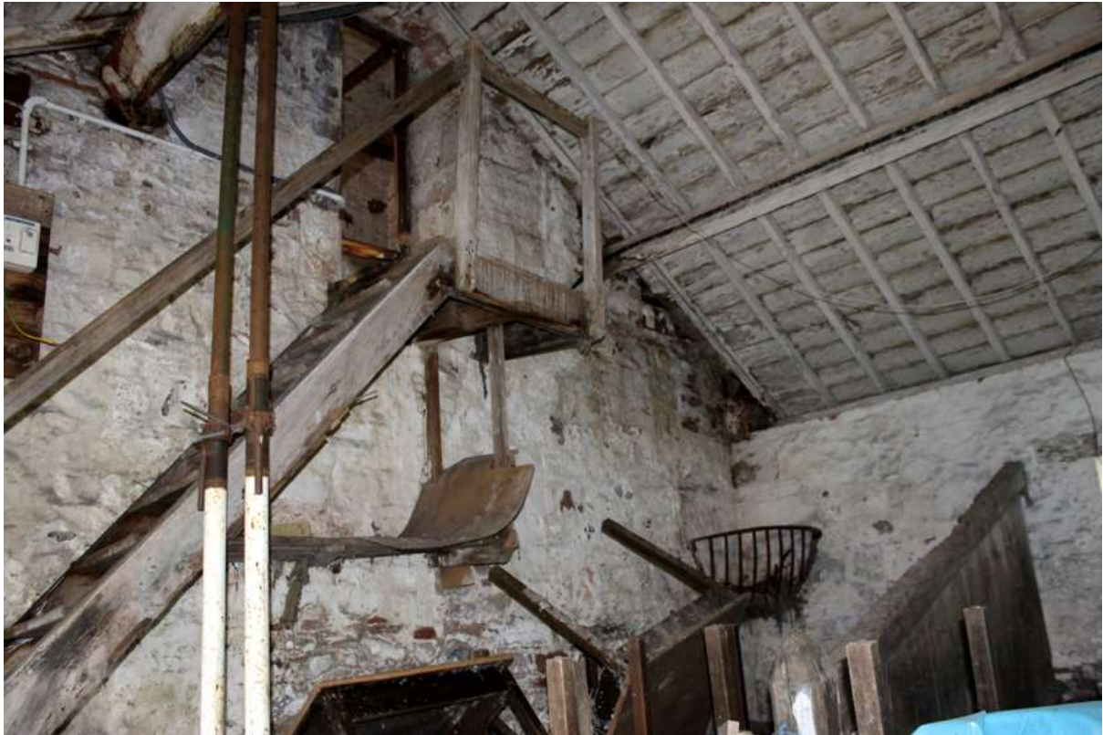
Fig. 22. East Wing – EW2 with stalls, feed boxes and stairs to tower,
