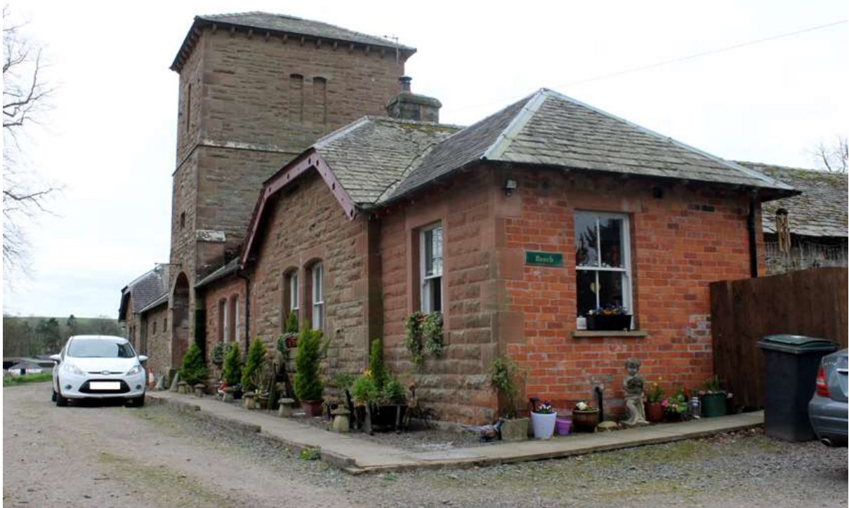
Fig. 22. East Wing – Beech Cottage showing modern bay with brick side wall.
