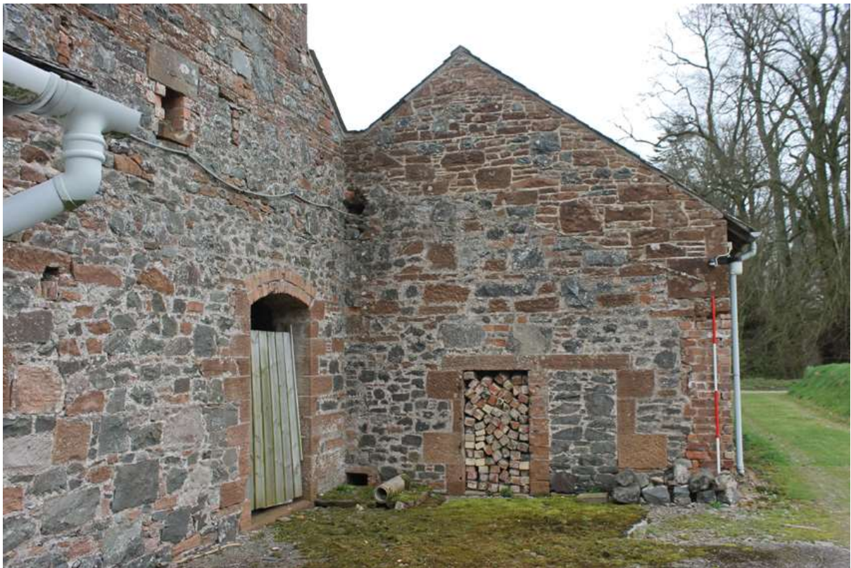
Fig. 15. South Wing – west gable.
