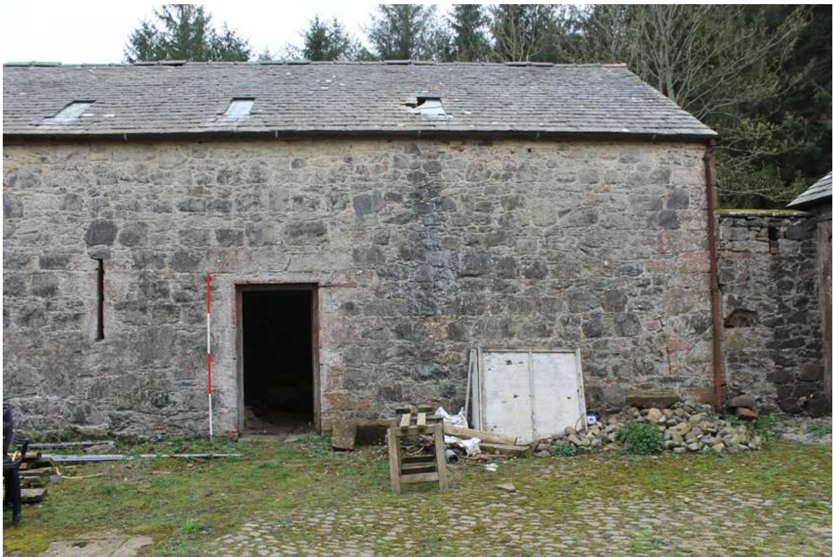
Fig. 7. West Wing – slit ventilator and entrance to WW1.
