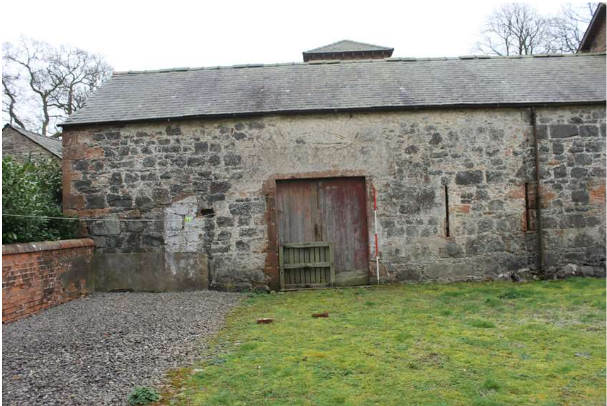
Fig. 9. West Wing – outer face of WW1 with cartway and slit ventilators.
