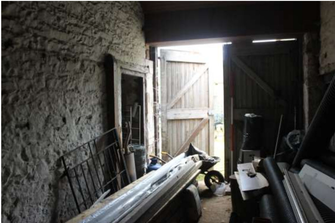
Fig. 15. West room showing door on left to main room.
