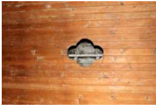
Fig. 13. Ceiling void for light fixture.
