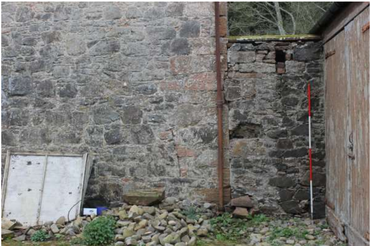
Fig. 7. Joining wall between west wing (left) and north wing (right).
