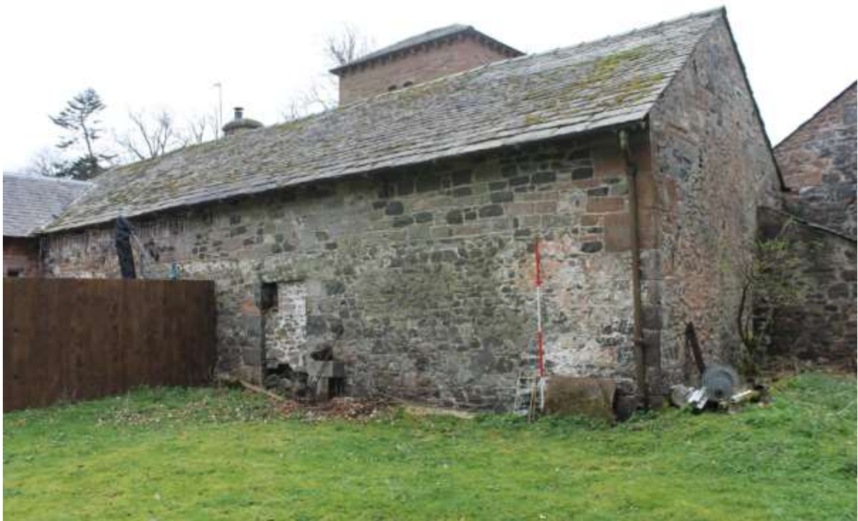
Fig. 9. North wall showing two-phase construction and blocked opening.
