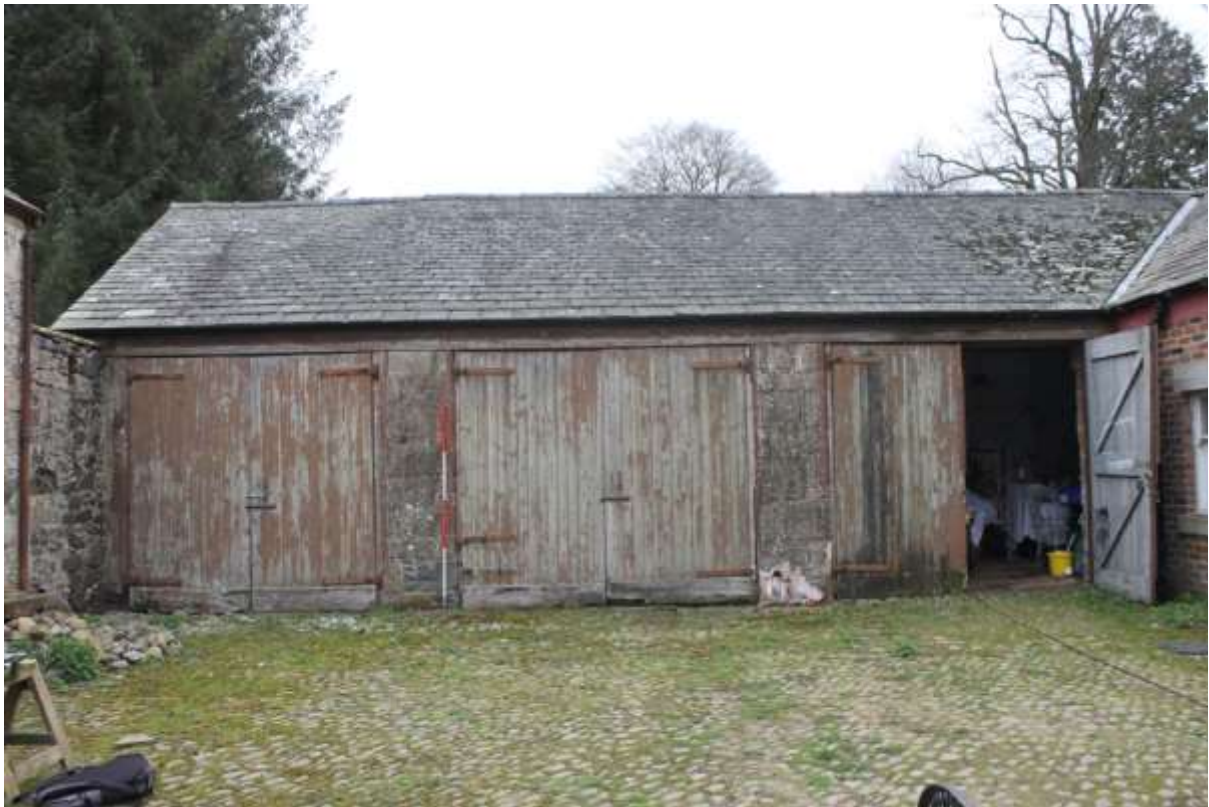
Fig. 6. South face of north wing.
