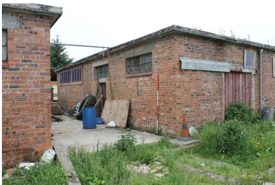
Fig.10. Building 1, NE corner.
