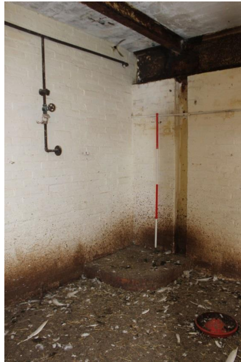
Fig.23. Building 2, plinth & heating pipes in 2f.
