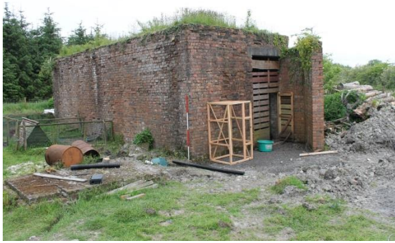
Fig.24. Building 3 from NE.
