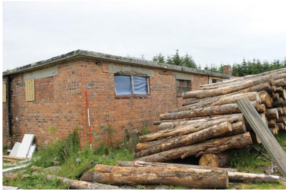
Fig.9. Building 1, NW corner.
