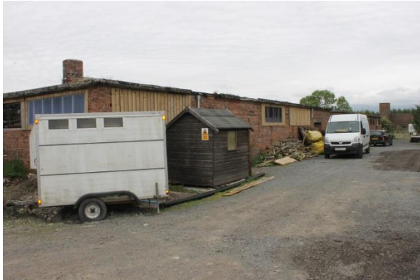
Fig.6. Building 1 from SW
