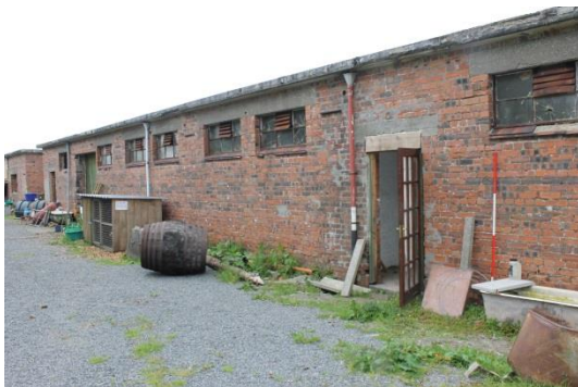
Fig. 16. Building 2 from SE.
