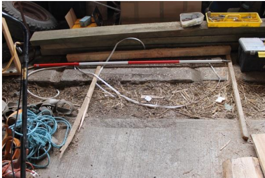
Fig. 14. Building 1, detail of drain.
