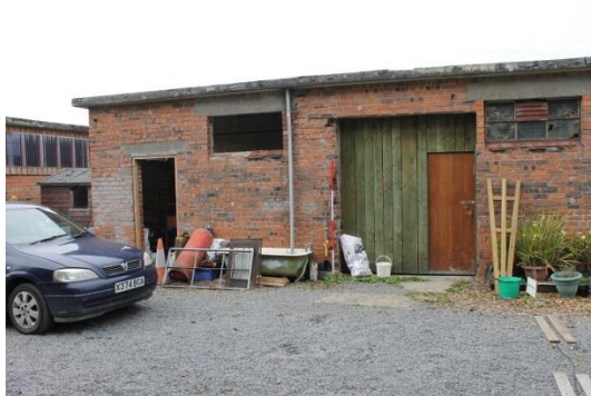
Fig. 17. Building 2, SW corner and entrance to 2b.
