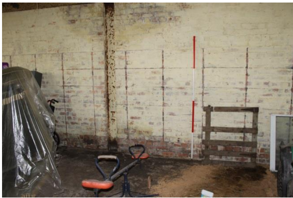
Fig.20. Building 2, E wall of 2a with outline of shelves.
