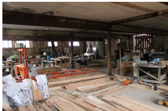
Fig.11. Building 1 interior from NW.
