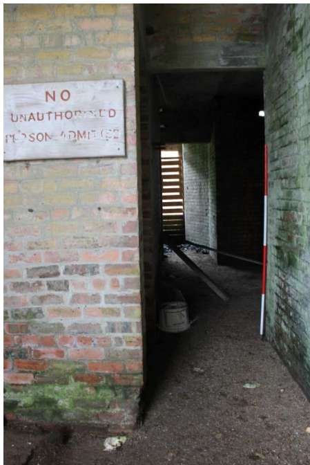
Fig.28. Building 3, N entrance passage.
