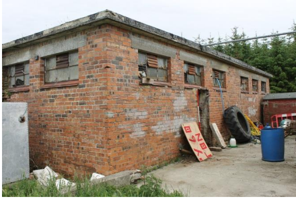
Fig.18. Building 2, NW corner.
