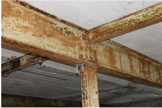
Fig. 12. Building 1, detail of RSJ construction.
