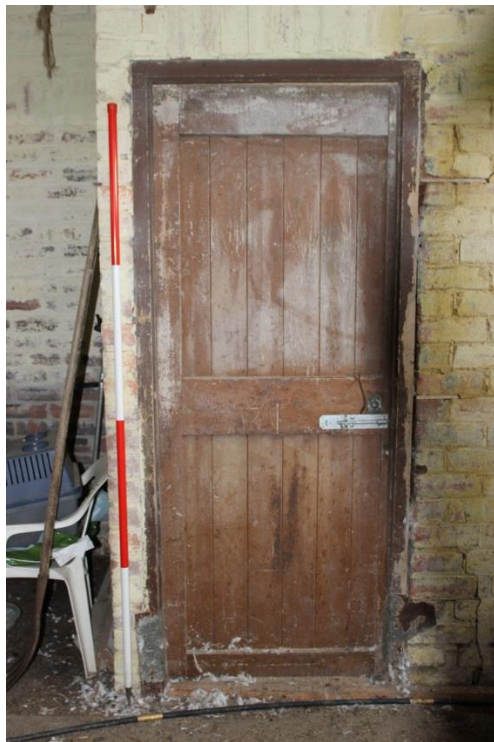
Fig.22. Building 2, original wooden door to 2d.
