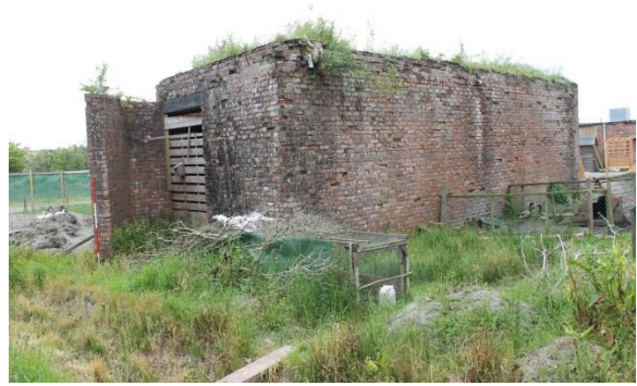
Fig.25. Building 3 from SE.
