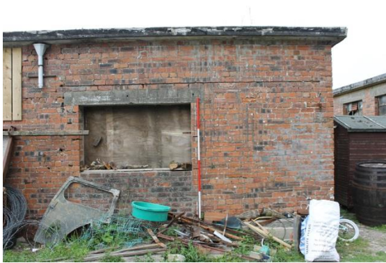
Fig.8. Building 1, blocked door, SE corner of S wall.
