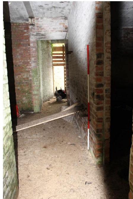
Fig.29. Interior looking N to entrance passage.
