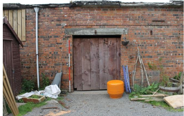
Fig.7. Building 1, main door on S wall.
