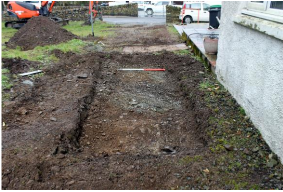
Fig. 12. Trench 2 from west.
