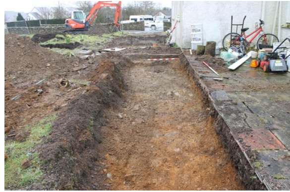
Fig. 8. Trench 1 from west.
