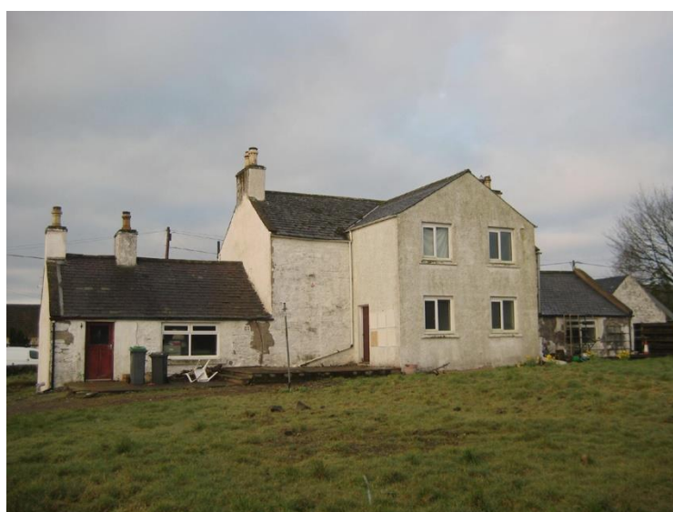
Fig.4. Pre-excavation view of the rear of Newhouse from the north-east showing the central extension.
