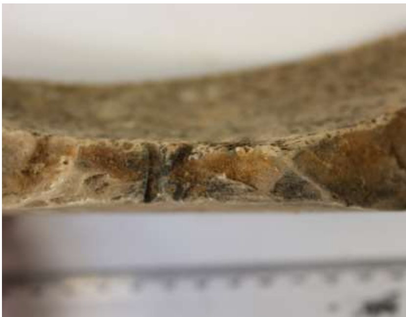
Figure 2: The riveted Mancetter-Hartshill base (Source: The Author)
