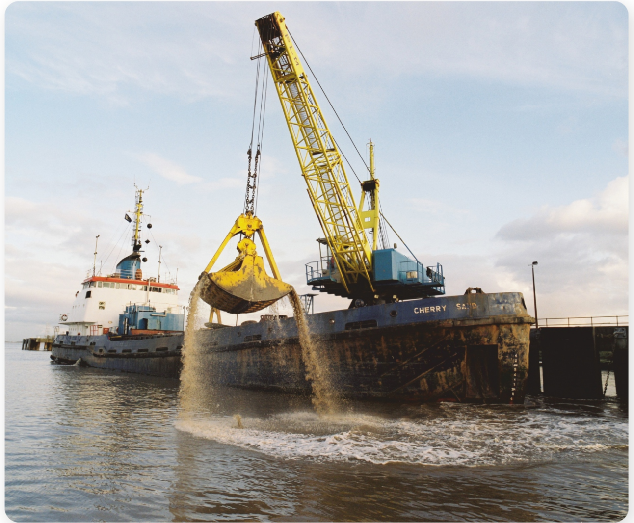
The grab dredger Cherry Sand in operation
