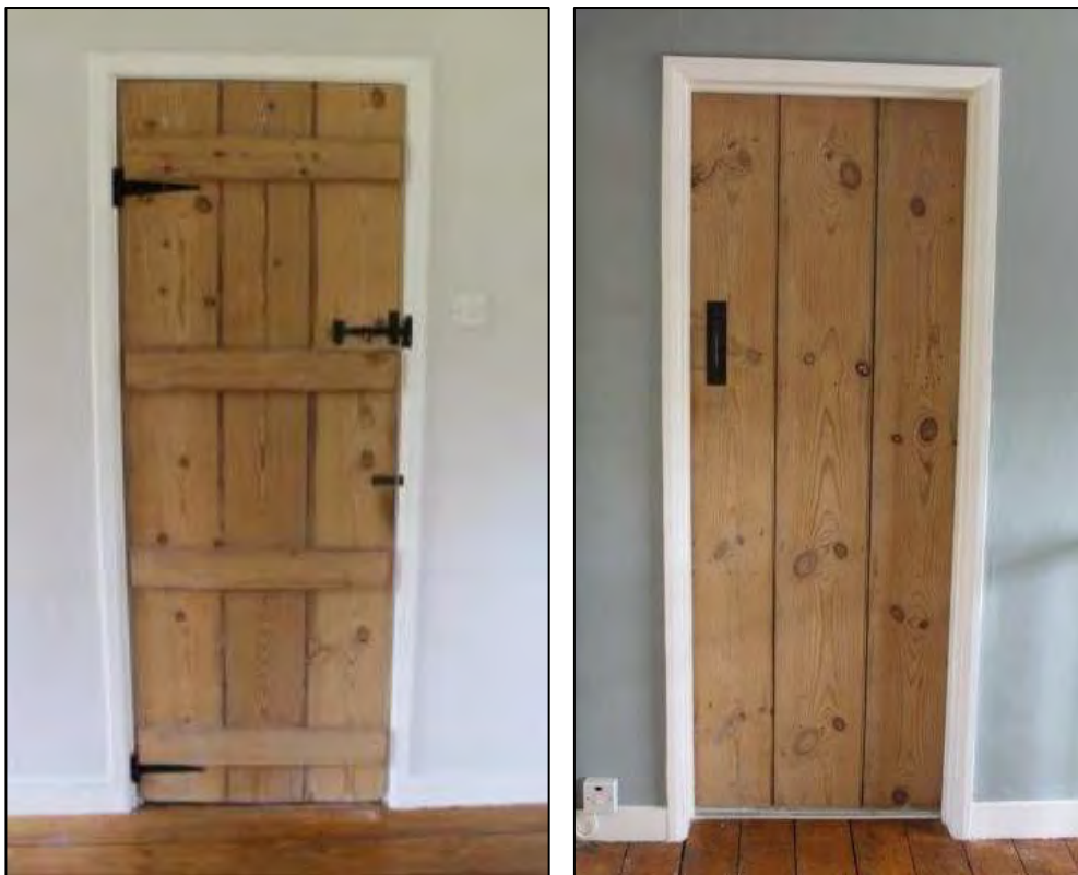
Photos 17 & 18 Braced and ledged doors used throughout the first floor
