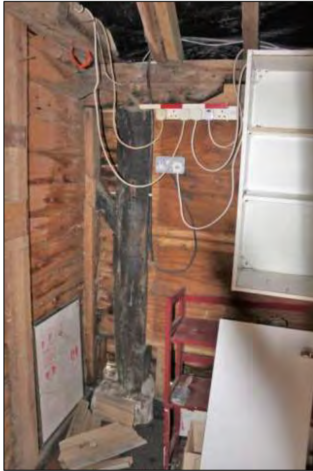
Photo 38 Detail of the south end of Frame C
