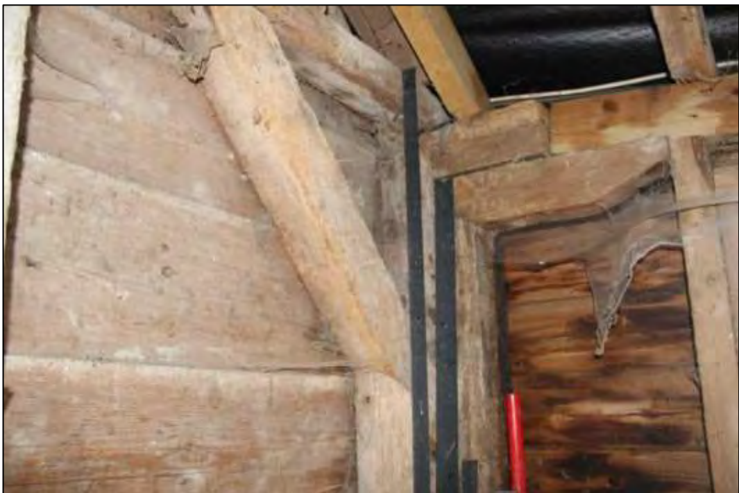
Photo 35 Detail of the south end of Frame B
