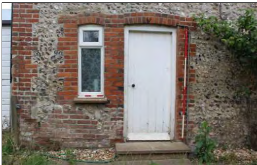
Photo 4 Detail of door and window in north elevation
