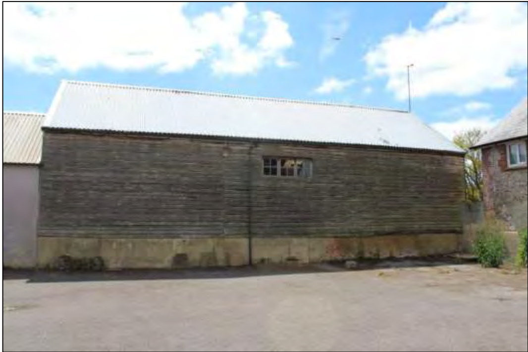
Photo 46 South elevation of the larger element of the Warehouse
