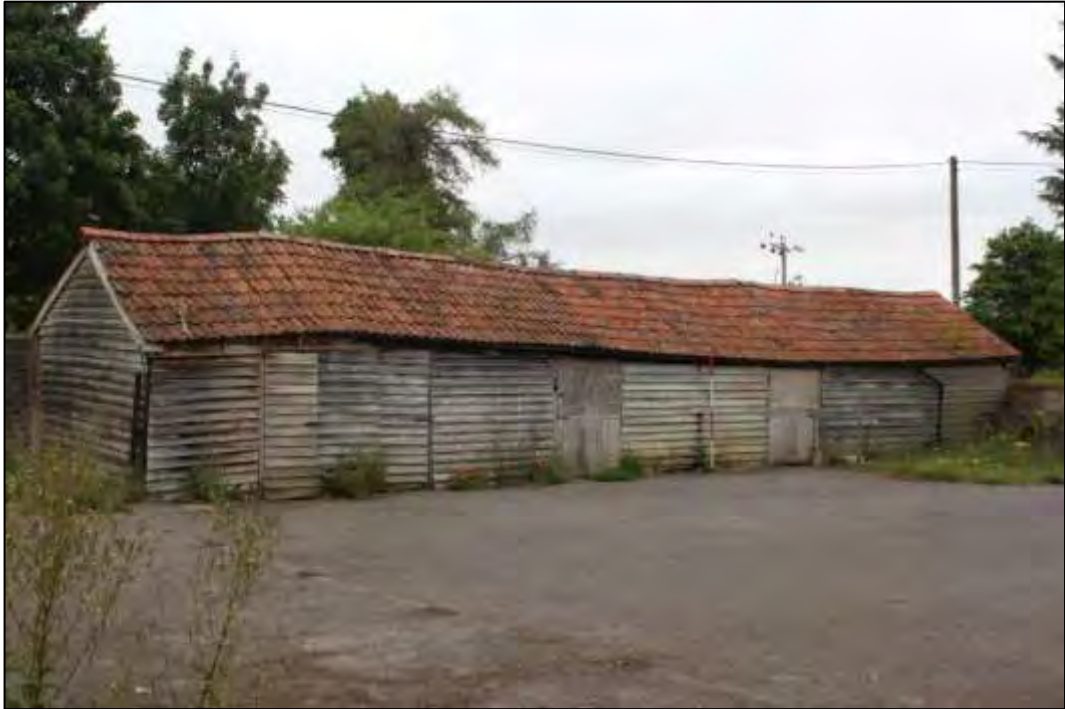
Photo 26 Shelter shed on the north side of the yard
