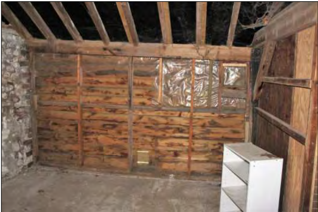
Photo 45 Internal view of infill to south elevation within Bay 6
