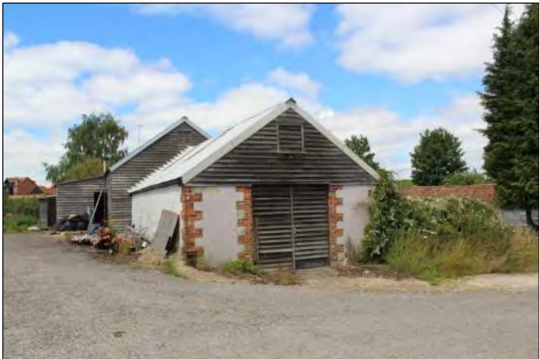
Photo 47 East elevations of the Warehouse
