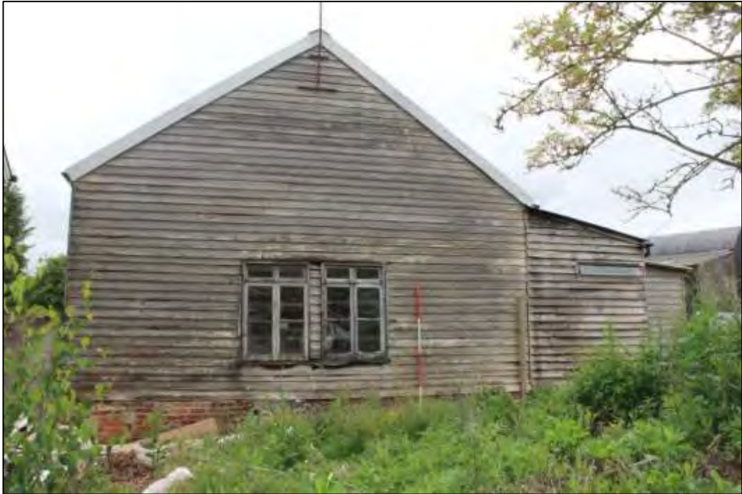
Photo 51 West elevation of the Warehouse's larger element
