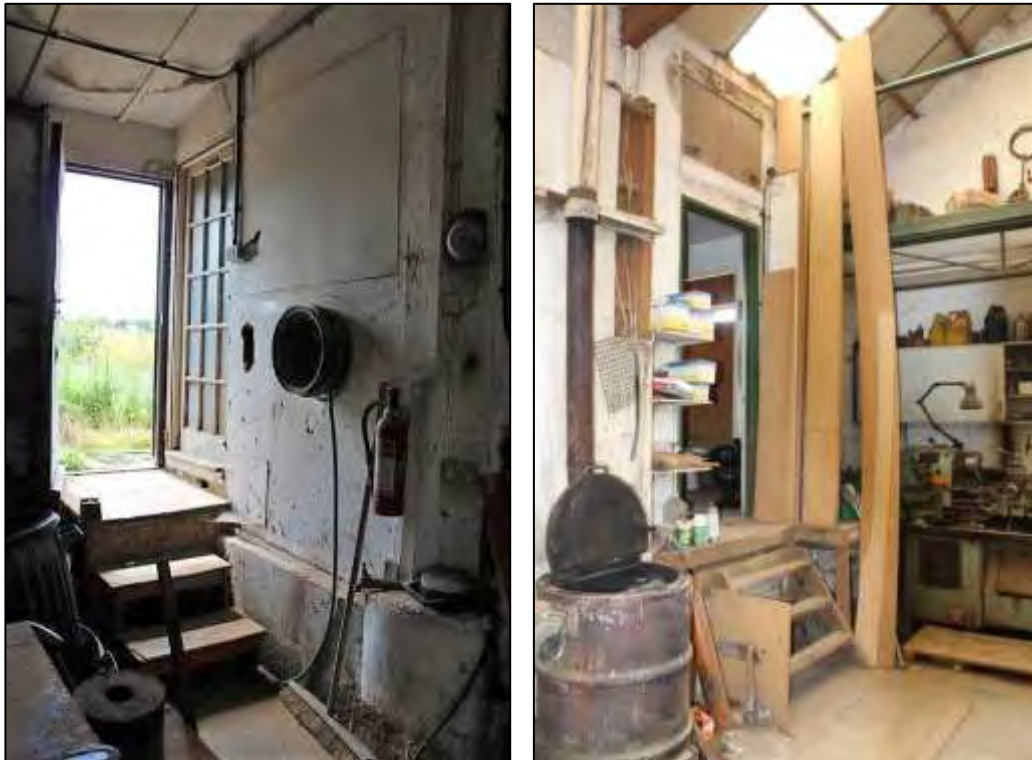
Photos 54 & 55 Access to the office from the main entrance (left) and to the kitchen from the workshop (right)
