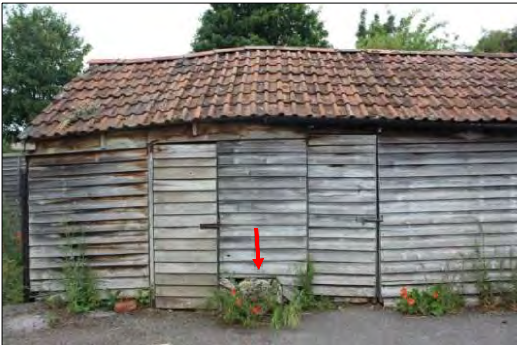
Photo 28 South elevation, with the padstone identified by the red arrow
