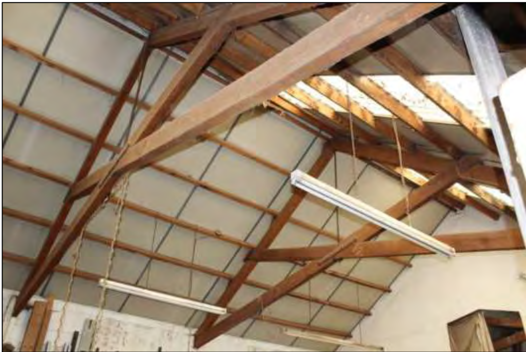
Photo 53 Scissor trusses in the larger Warehouse element
