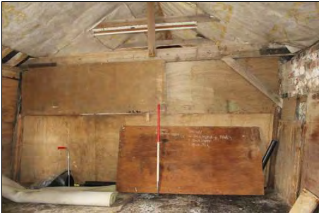
Photo 43 Partition on Frame D
