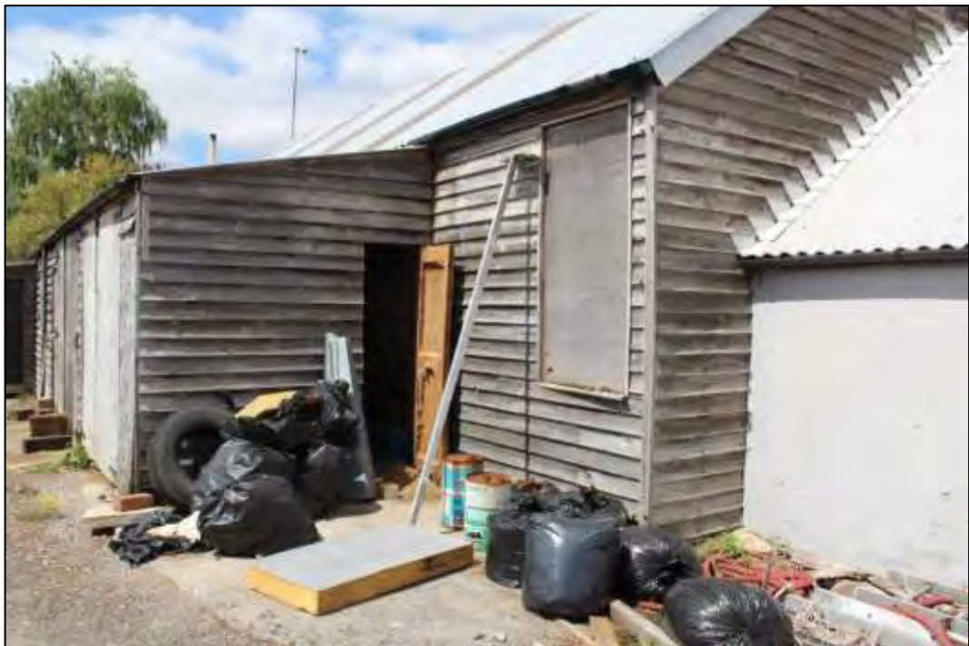
Photo 50 South-east corner of the Warehouse's larger element
