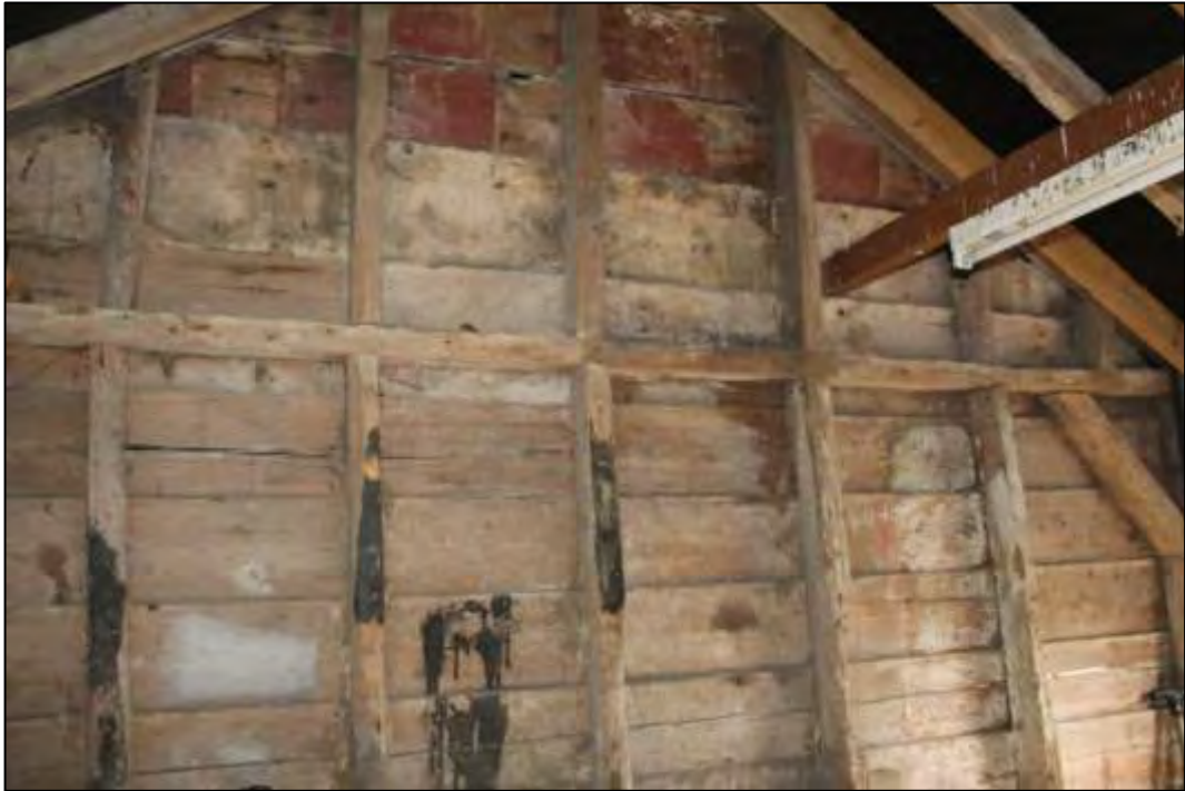
Photo 33 South face of Frame B, between Bays 1 and 2
