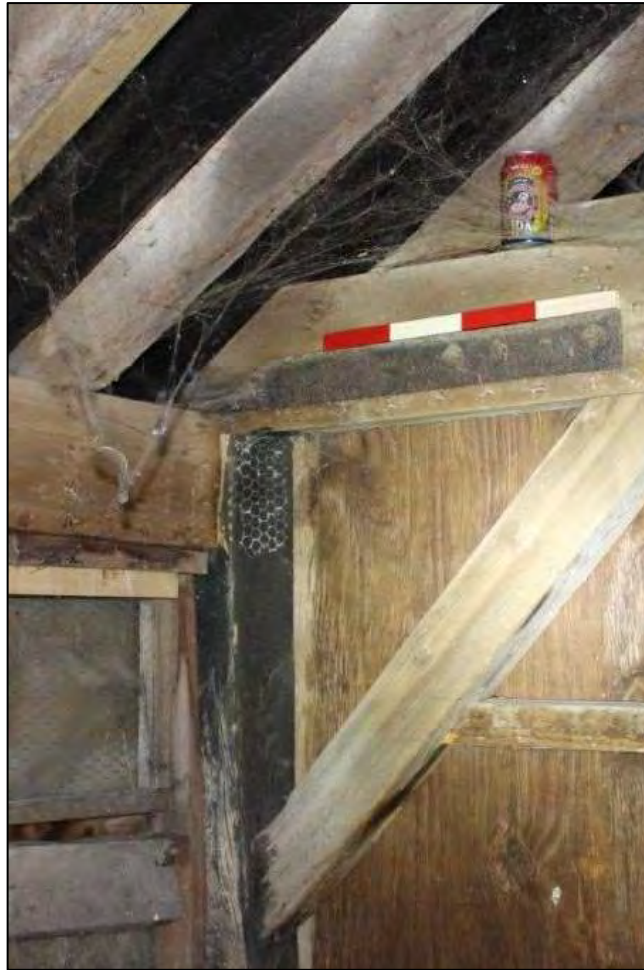
Photo 42 Post on Frame F
