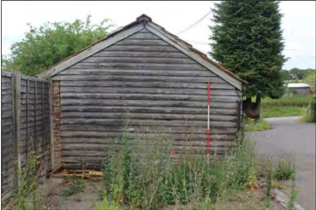
Photo 27 West end of the shelter shed
