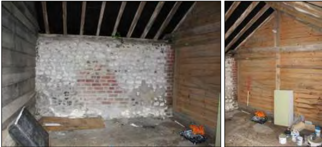
Photos 36 and 37 North (left) and east (right) walls within Bay 2
