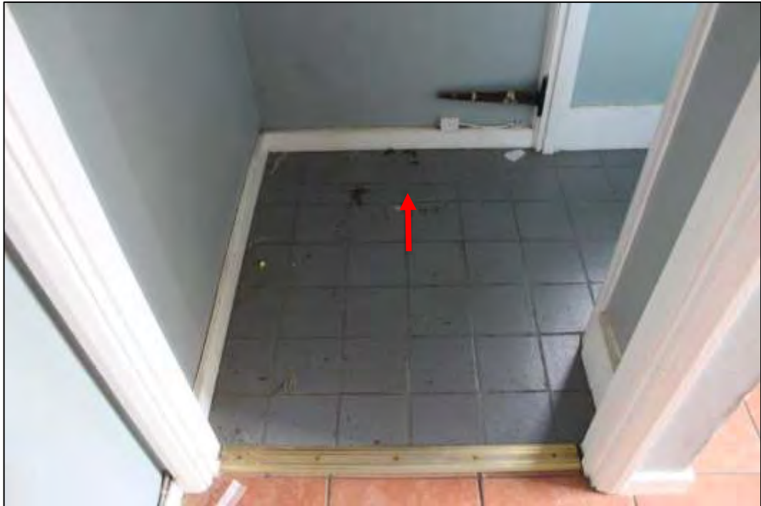
Photo 10 Lobby to WC, with stone threshold indicated by red arrow
