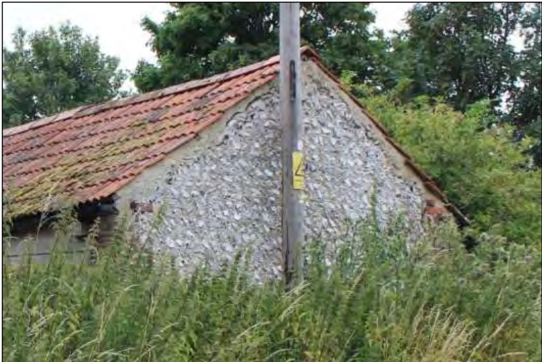
Photo 31 East elevation of the shelter shed
