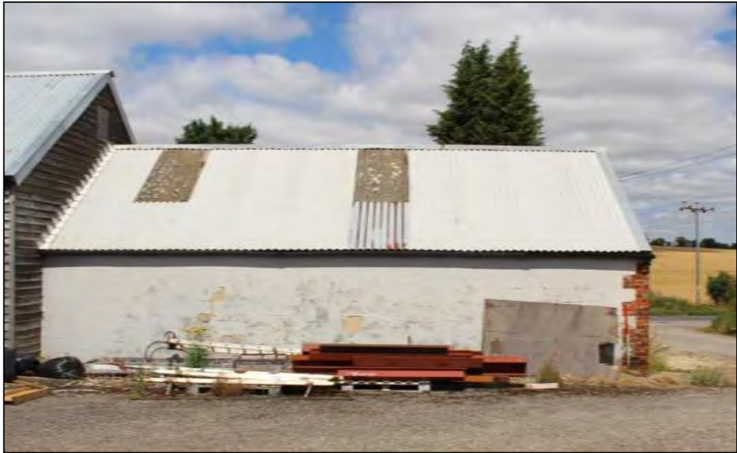
Photo 48 South elevation of the Warehouse's smaller element
