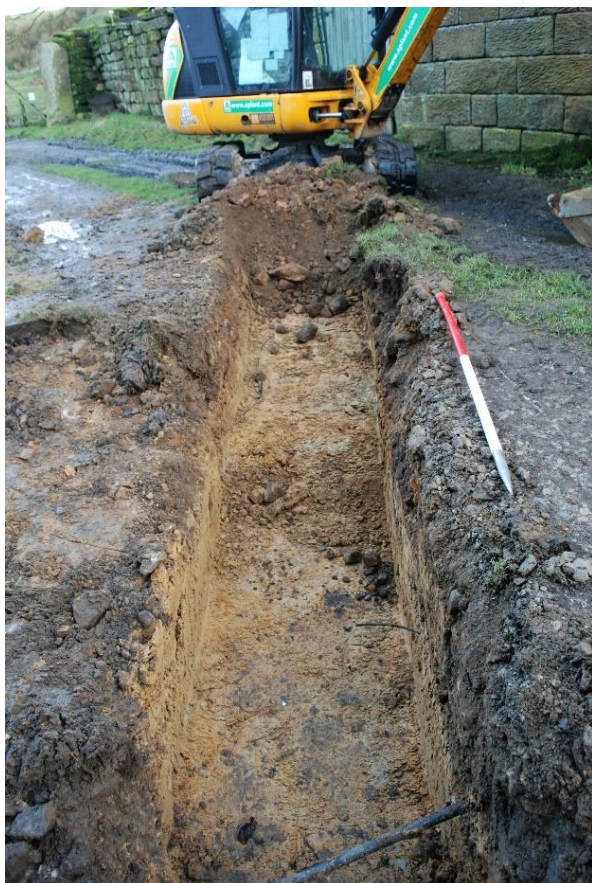
Plate 1: Overall shot of service trench. Facing north-east.
