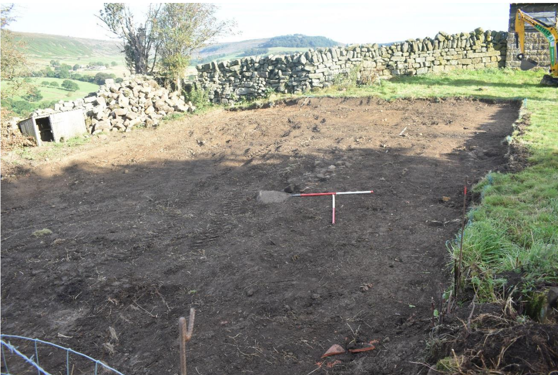
Plate 8: Watching brief stripped area of proposed car park area. Facing west.
