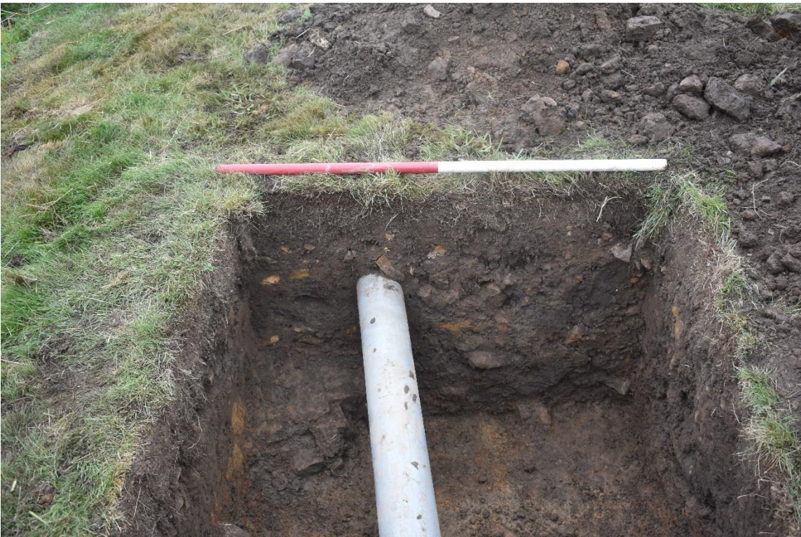
Plate 6: Test Pit 5. South – facing section 3 of service trench [5/005]. Facing north.
