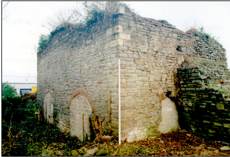
Figure 2.28: Exterior of pot arch building {15}/{16}, from west.
