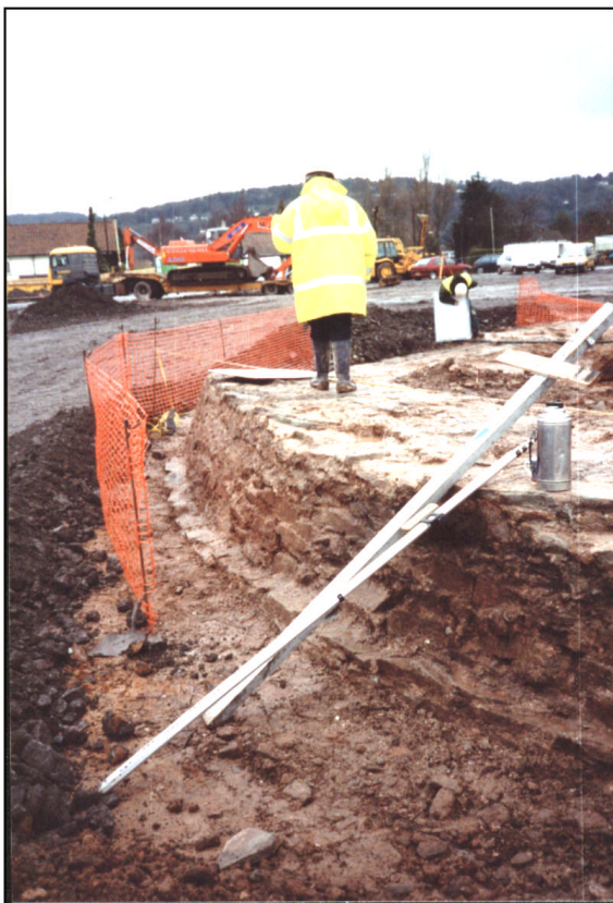
Figure 2.48: New House Cone, showing foundation extension - western sector
