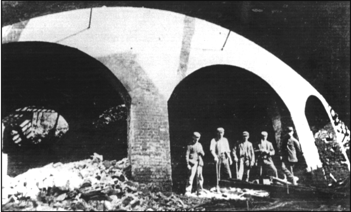
Figure 2.8: The Nailsea Glassworks Cone Supports, revealed during demolition in 1905 (NDLHS)
