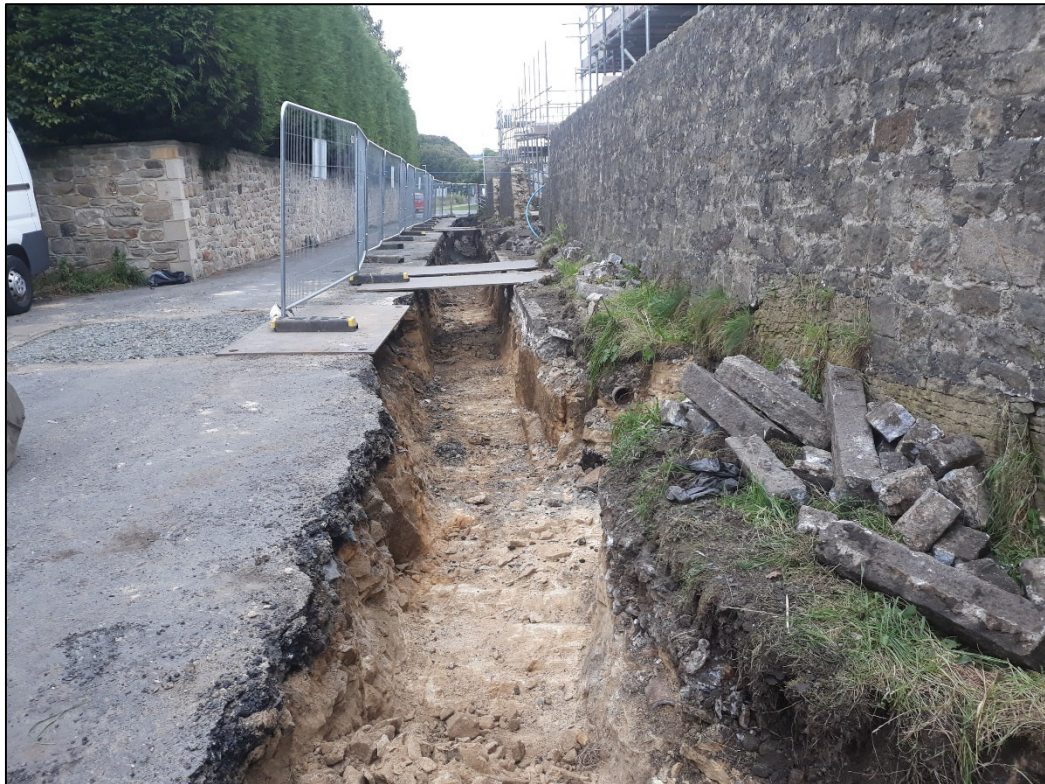
Plate 13; Western end of service trench within military road showing bedrock (1002)
