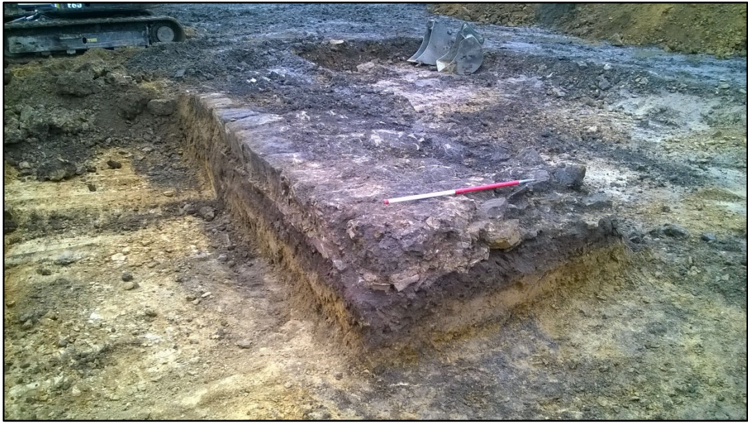
Plate 5; Hadrian's Wall foundations ( 109 ) including base stones ( 115 ), 1x 1.0m scale
