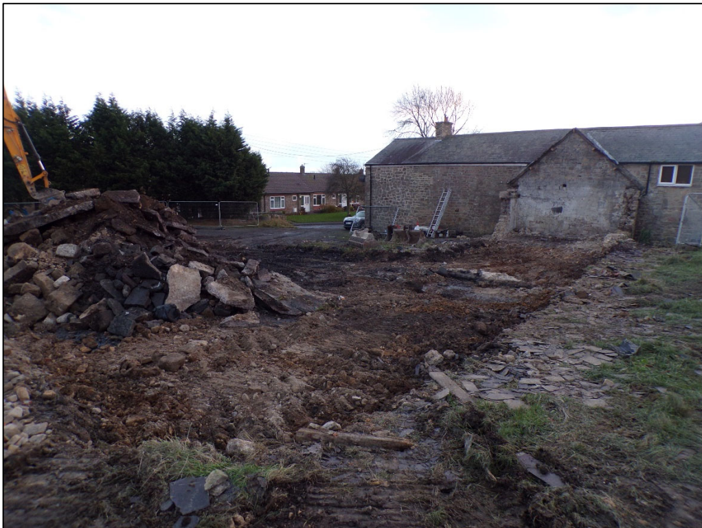
Plate 2; Site clearance works and levelling of site
