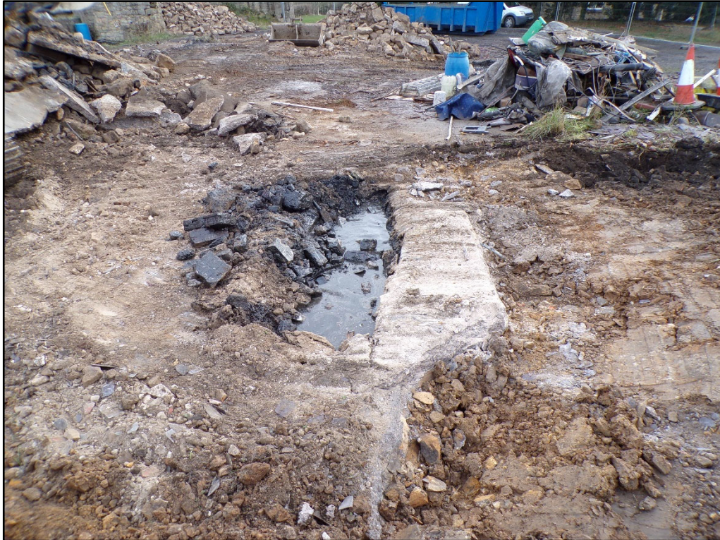
Plate 1; Site clearance works showing concrete foundations
