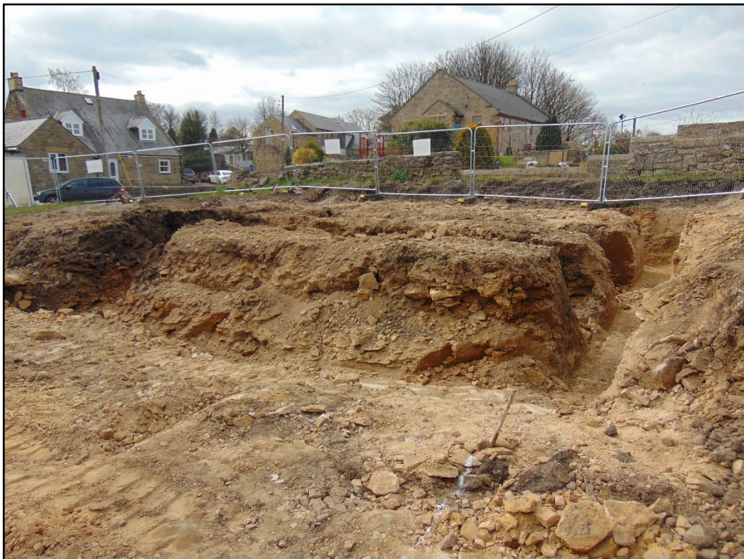
Plate 12; Foundations showing sandstone bedrock (108)
