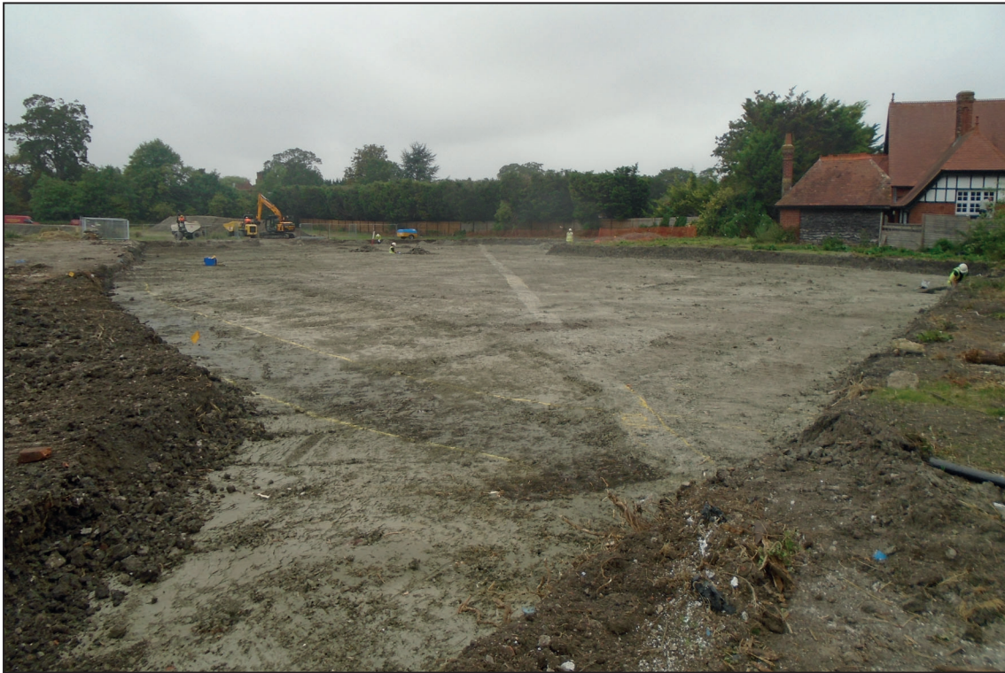
Overall site photograph, looking west
