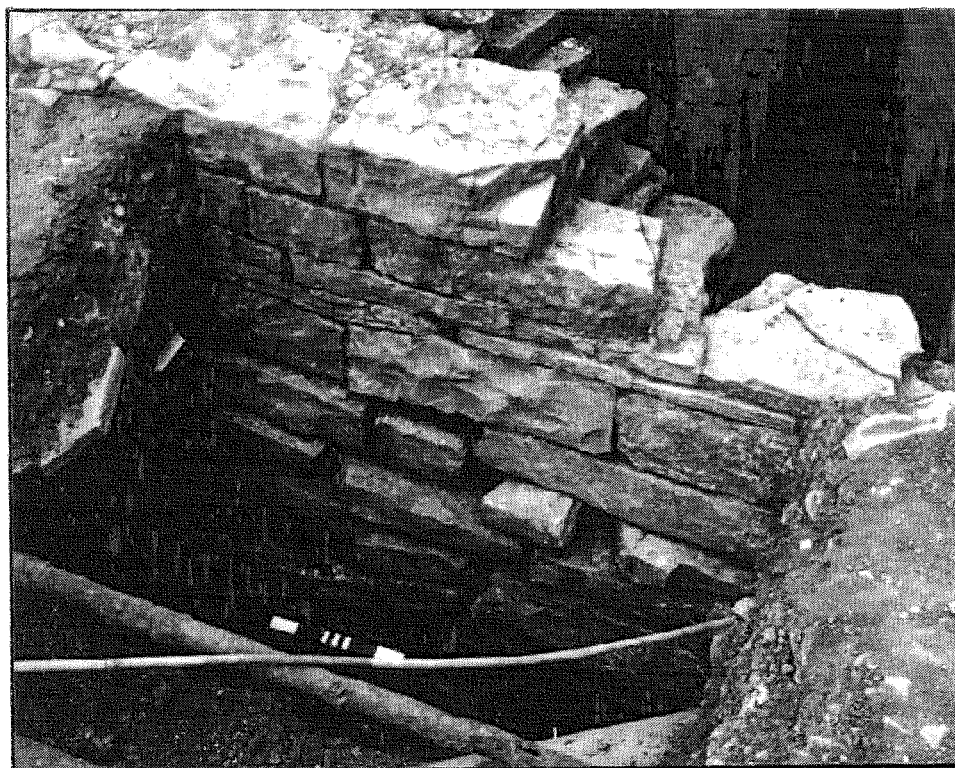
Figure 8: Photograph of elevation of Abbot Chryton's Wall
