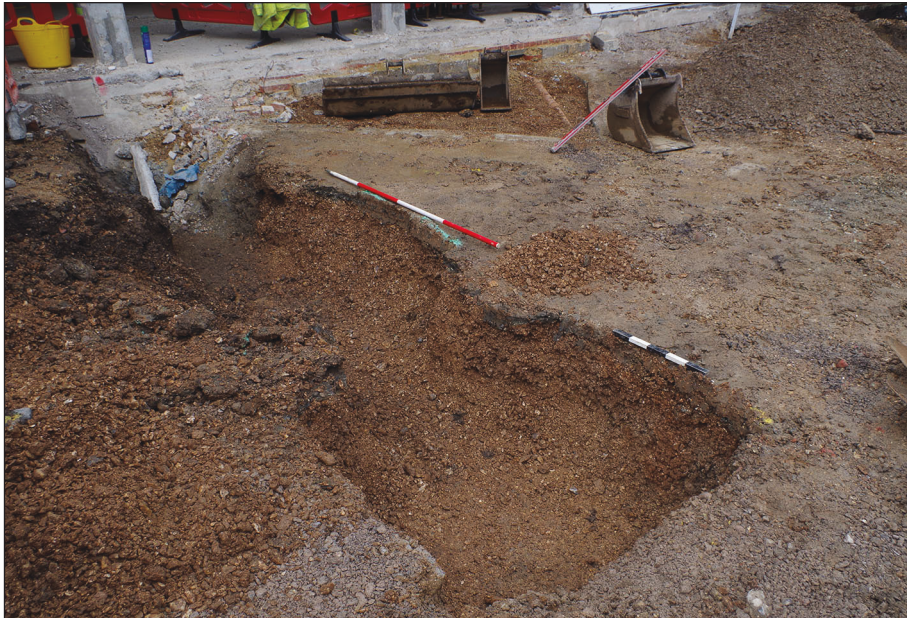
Plate 2: Trench 12 foundations viewed from the east. Scales are 2 m and 0.5 m
