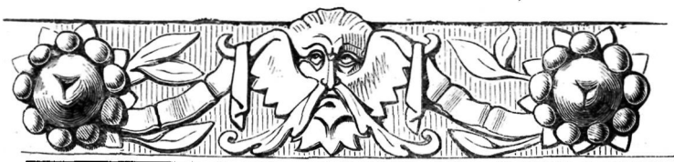
Cornice at No. 18, Bishopsgate Street Without.
