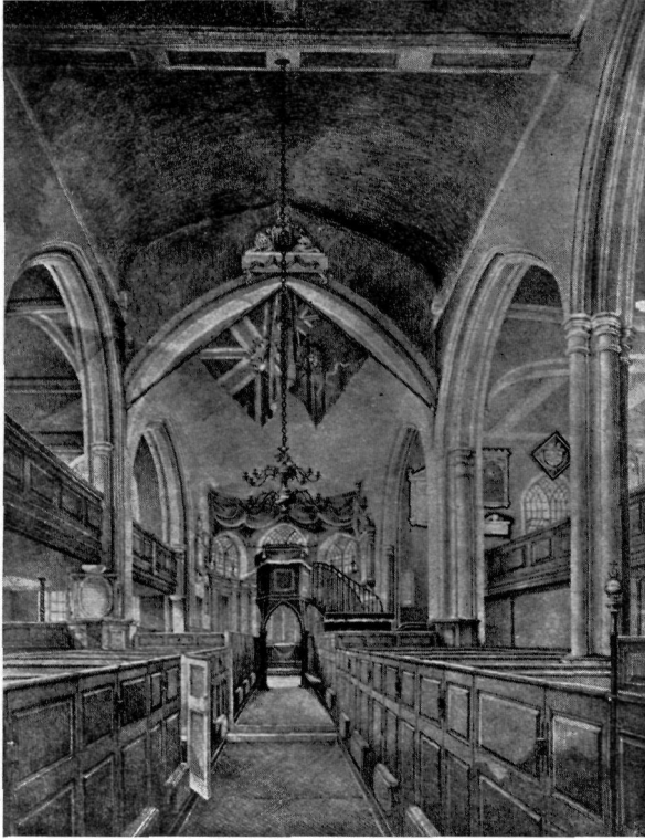
INTERIOR, LOOKING EAST. (Prosser, 1827.)
