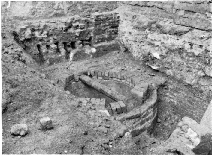
9. THE WELL AND WELL CHAMBER. Partly uncovered
