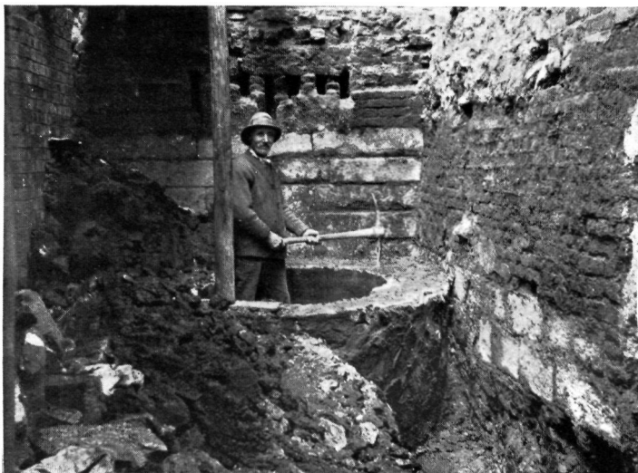
15. GENERAL VIEW OF WELL, WELL CHAMBER AND RETAINING WALL.
