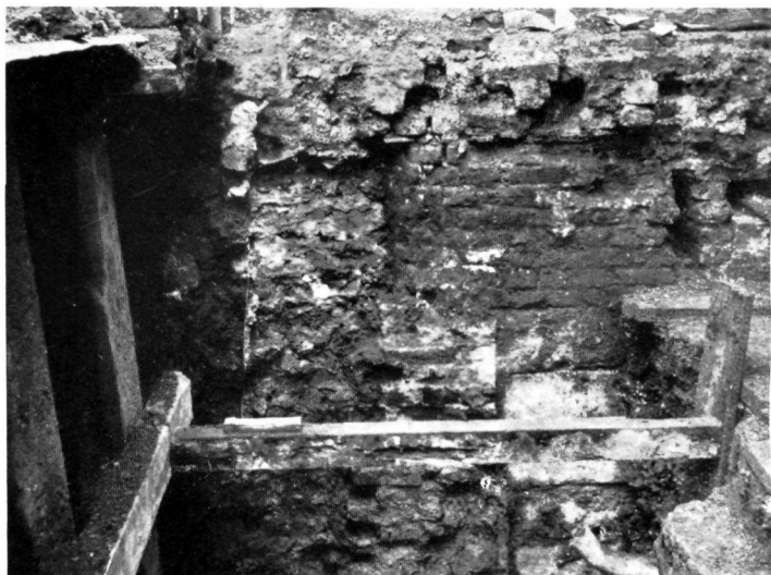
11. NORTH WALL OF WELL CHAMBER, SHOWING ROUNDED ANGLE.
