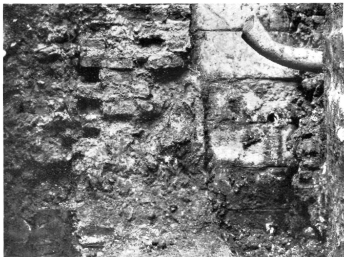
12. N. END OF WELL CHAMBER, WITH PIPE FROM CIRCULAR WELL.
