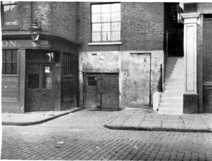
6. STEPS FORMERLY LEADING TO RAY STREET PLACE.
