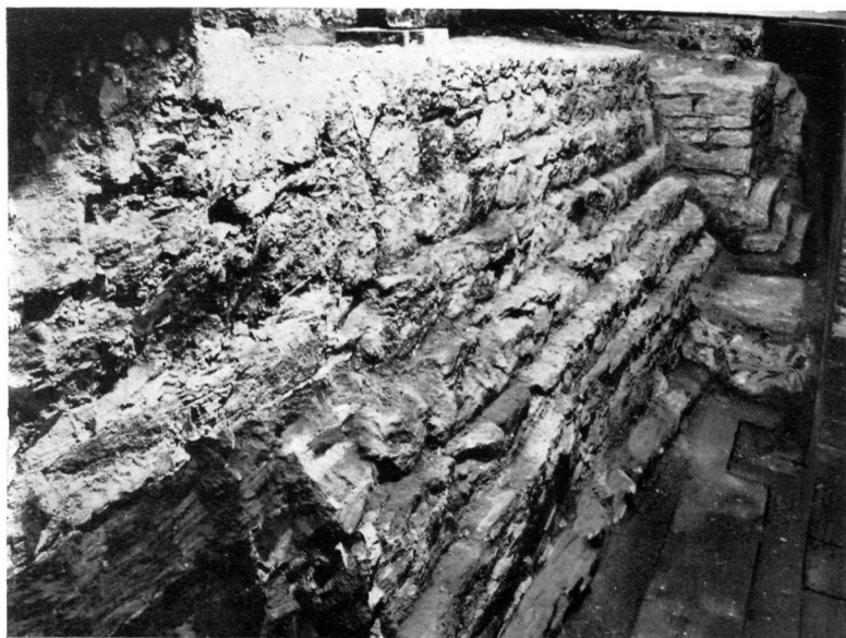
Fig. 4.—EASTERN END OF RAGSTONE WALLING RUNNING FROM THE NORTH WALL OF THE SERVANTS' HALL OF THE PRIVATE HOUSE OF THE OFFICES OF THE TIMES .
