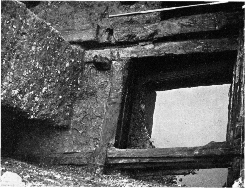
Plate 1.—Custom House site; Trench III, Roman quay looking south (scale in 0.5 m.)
