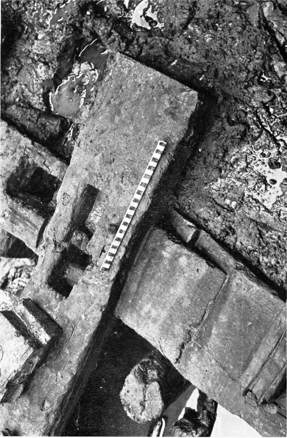
Plate 3. Custom House Site. "Trait-de-Jupiter" scarf joint from the ground plate of the second period medieval waterfront. (Scale in cms.).
