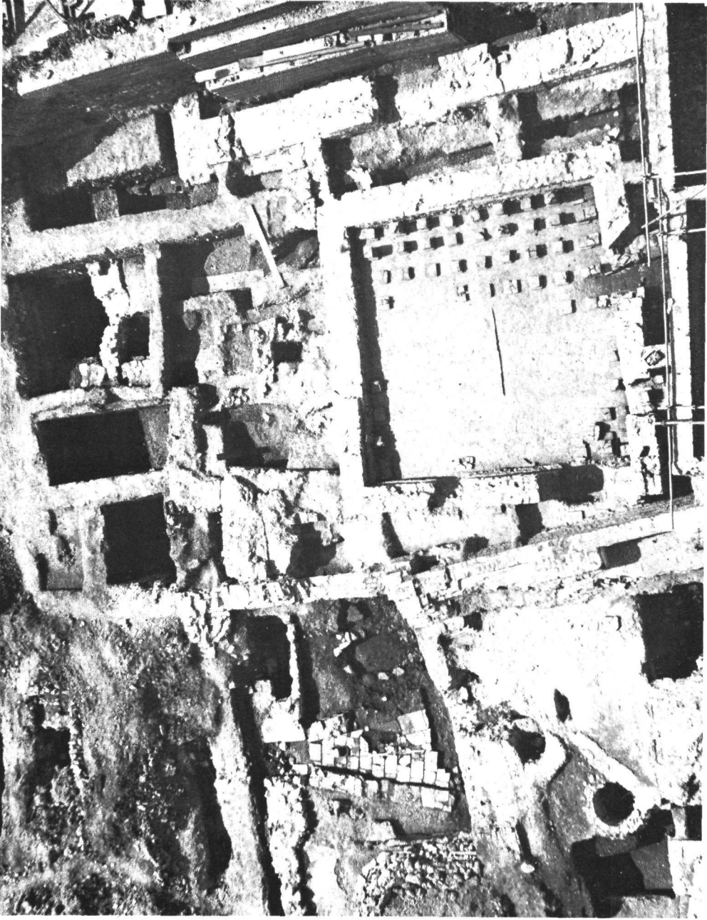
Plate 3. Huggin Hill baths: The eastern part of the baths viewed from the north, showing the square Room 30, and on its right the corridor 29. The caldarium , Room 33, is on the left. Scale of feet.
