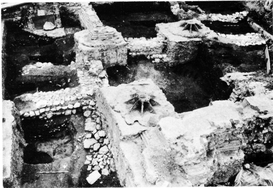
Plate 15. Milk Street: early medieval undercroft foundations, looking S.
