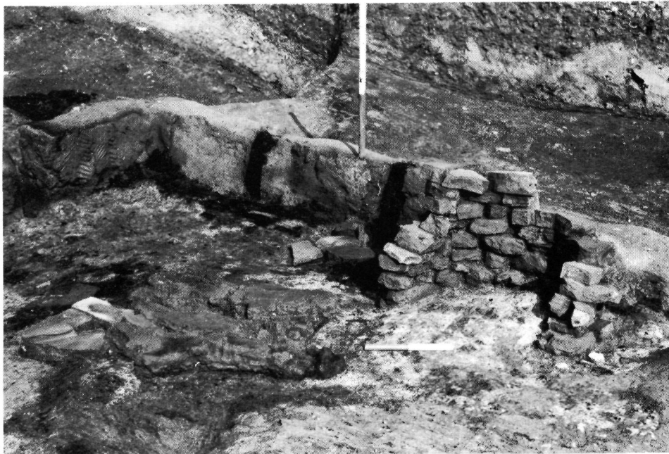
Plate 5. GPO Newgate Street: interior of early 2nd-century Roman building, showing domestic hearth with ash spread (right), burnt studs of timber framework (middle) and chevron internal wall decoration (left).
