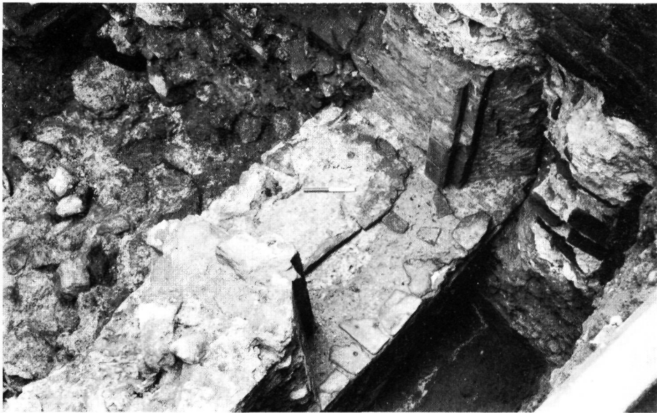
Plate 18. Duke's Place: medieval doorway inserted into the city wall, probably by the adjacent Holy Trinity Priory, 13th or 14th century.
