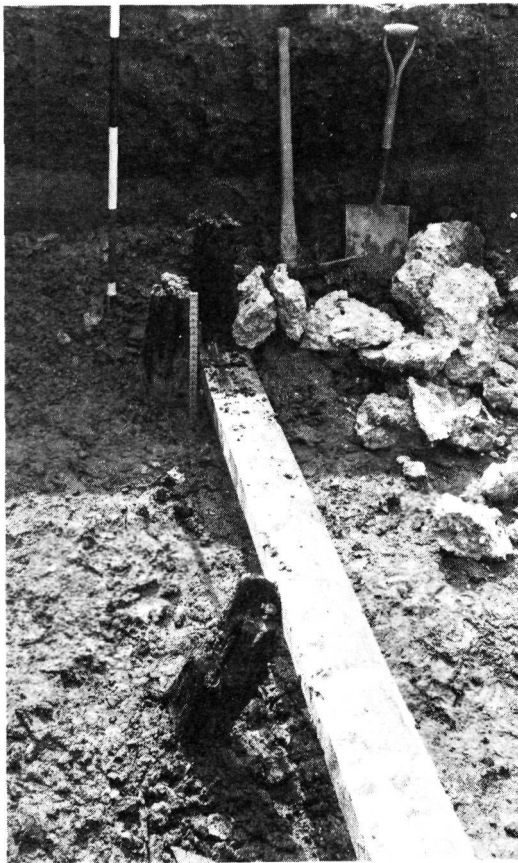
Plate 1. Queen Street, 1953 & 1960: Timber piles, Feature 21.
