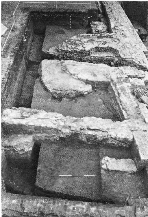
Plate 10. Eltham Palace: The east front of the range of queen's apartments, and the tower at the north-west corner of Henry VIII's chapel, showing the well of the stair (Photo: Derek Craig).
