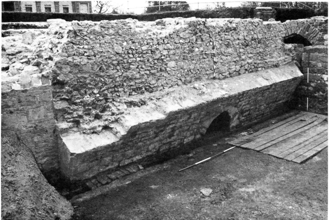
Plate 4. Eltham Palace: Detail of south wall of Bishop Bek's cellar, showing the change in vaulting (left) at the east end, the central relieving arch, and (next to the far ranging pole) the ventilation shaft ( Photo: Derek Craig ).
