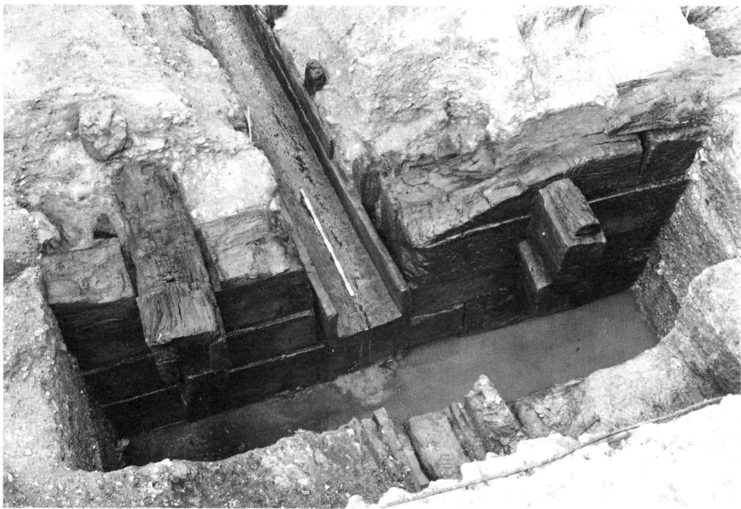
Plate 2. Pudding Lane Excavation, Area C. Late 1st-century timber-faced quay; looking north; low tide. 10 × 100mm scale rests in dugout drain set in facing of quay between protruding heads of tiebacks. River level at Ordnance Datum.
