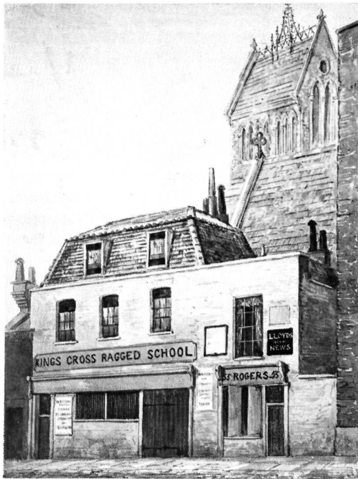
2. Kings Cross Ragged School, Britannia Street, c. 1865.
