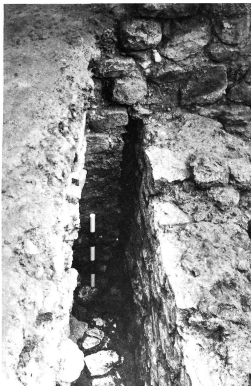
Plate 9 Water Lane 1977: Abutment of Roman riverside walls viewed from west. North (landward) face of 3rd-century wall to right, southern extension of late 4th-century wall behind ranging rod; 13th-century curtain overrides junction (1m scale).
