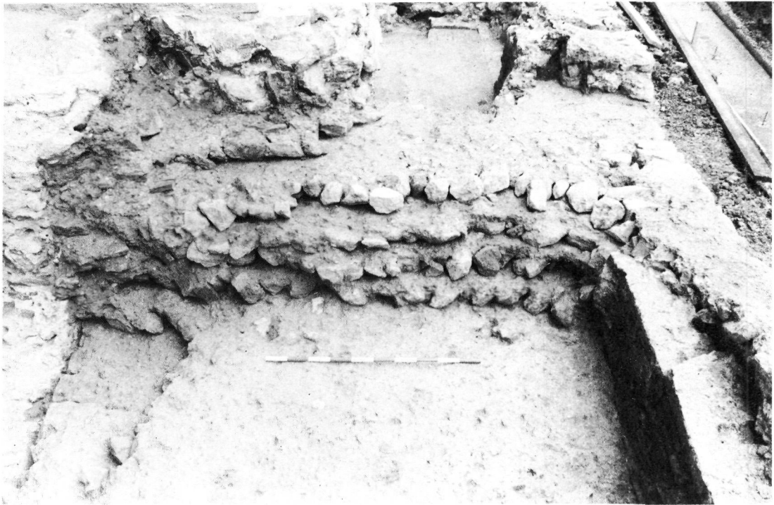
Plate 6 Inmost Ward 1977: Core of late 4th-century riverside wall revealed by removal of lining of post-medieval brick cellar. South face of wall and later medieval addition far left (1m scale).
