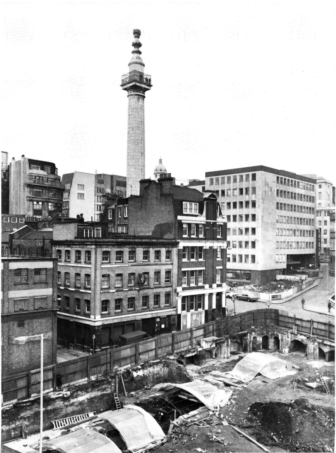
Fig. 1 Pudding Lane: Excavating on the Peninsular House site, Pudding Lane, in the shadow of the Monument. The polythene cover on Area B has been rolled back revealing the cellar of a building burnt in the Great Fire of London.
