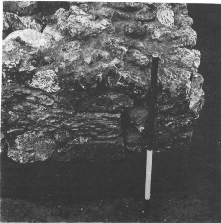
Plate 7. Close up of the junction of walls F7 and F24 (looking south), showing the continuation of rebuild F114 over F24.
