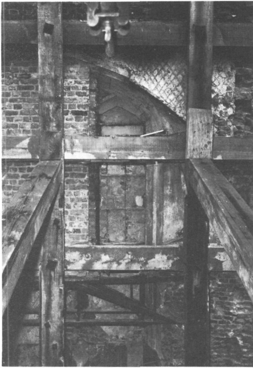
Plate 9 Whitehall: Great Close Tennis Play, remains of exterior of window in west wall II.T.4 (Crown Copyright)
