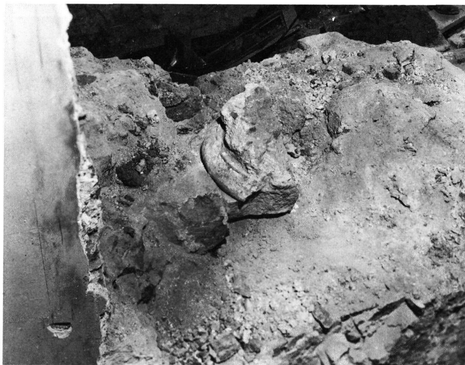
Plate 5 Whitehall: Great Close Tennis Play, south wall II.T.2, showing re-used medieval stonework in rubble core of Tudor wall (Crown Copyright)
