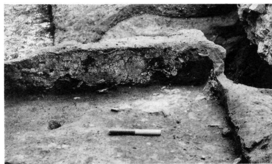
Fig 34. Building 6, Leadenhall Court site (LCT84): traces of plaster rendering on internal face of brickearth wall
