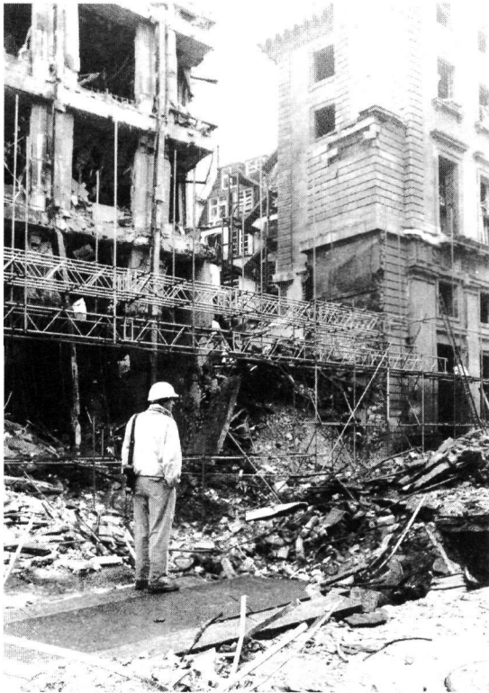
Fig 65. St Ethelburga Bishopsgate (38): view of the church shortly after the bomb blast of April 1993. The west wall had fallen into Bishopsgate
