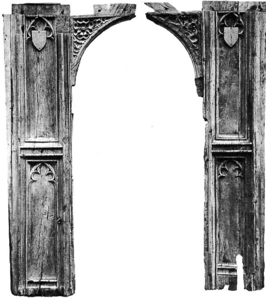
Fig 33. St Ethelburga Bishopsgate (38): 15th-century partition forming the doorway within the western entrance, now in the Museum of London
