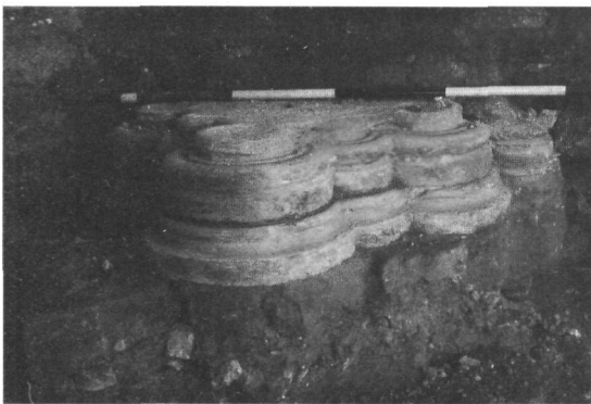
Fig 79. St Mary le Bow (69): 13th-century pier base found in 1955, re-used in post-Fire building works in the crypt. Scale is in feet (GM)
