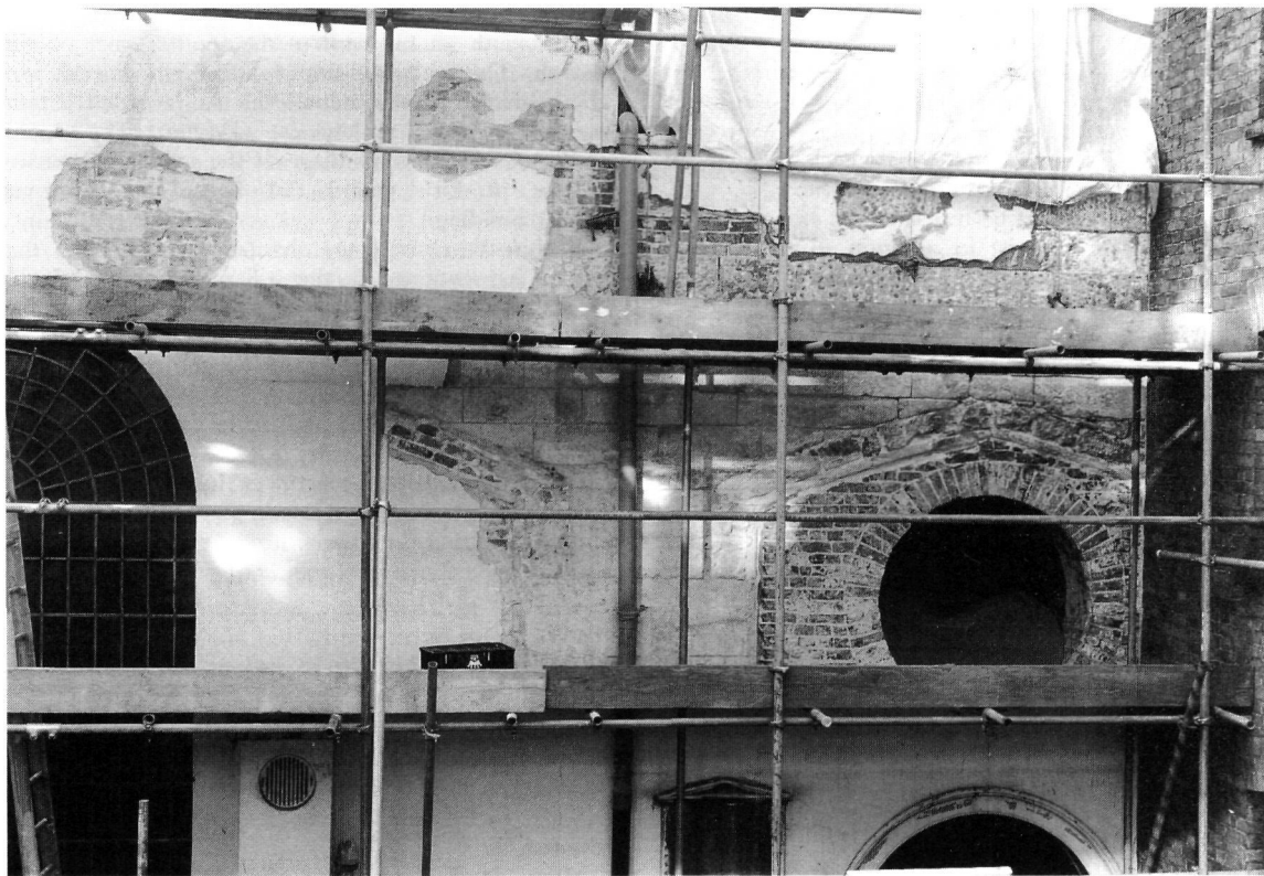
Fig 80. St Mary at Hill (71): the north aisle of 1497–1503, partially revealed within the Wren structure in 1984
