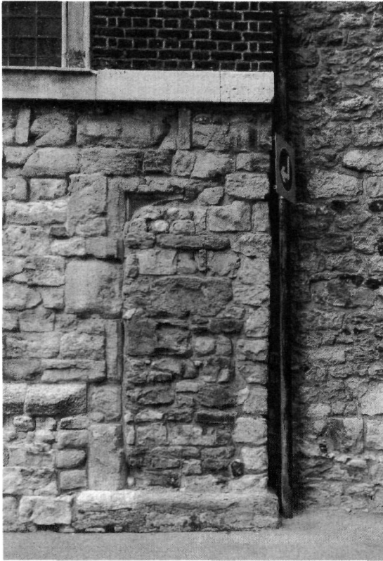
Fig 92. St Vedast Foster Lane (108) : south door to nave, revealed in 1992–3 after removal of rendering
