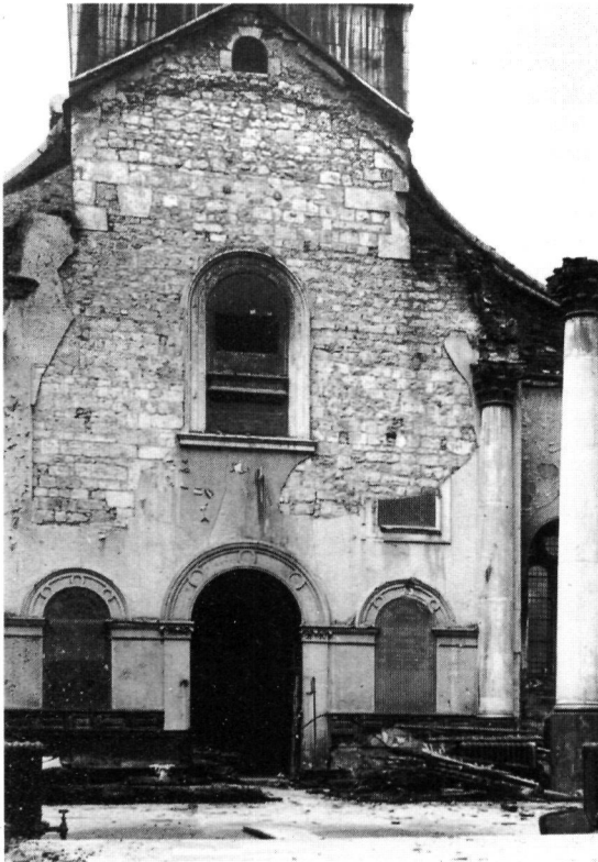
Fig 78. St Mary Aldermanbury (65): the west end of the Wren church, before removal to the USA. It is probable that much of this facade was of pre-Fire origin (GM)
