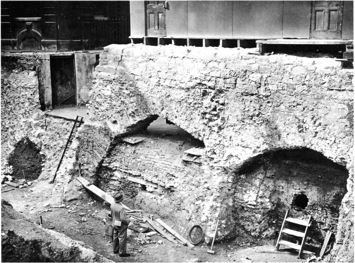
Fig 52. All Hallows Lombard Street (6): arches of the north arcade uncovered during demolition in 1939 (GM)
