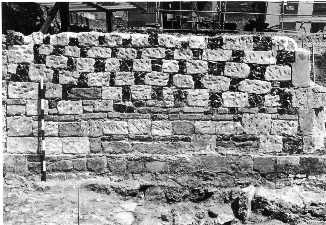
Fig 34. St Botolph Billingsgate (29) : chequerwork on the interior of the east wall of the south aisle or chapel, recorded on the Billingsgate Lorry Park site in 1982
