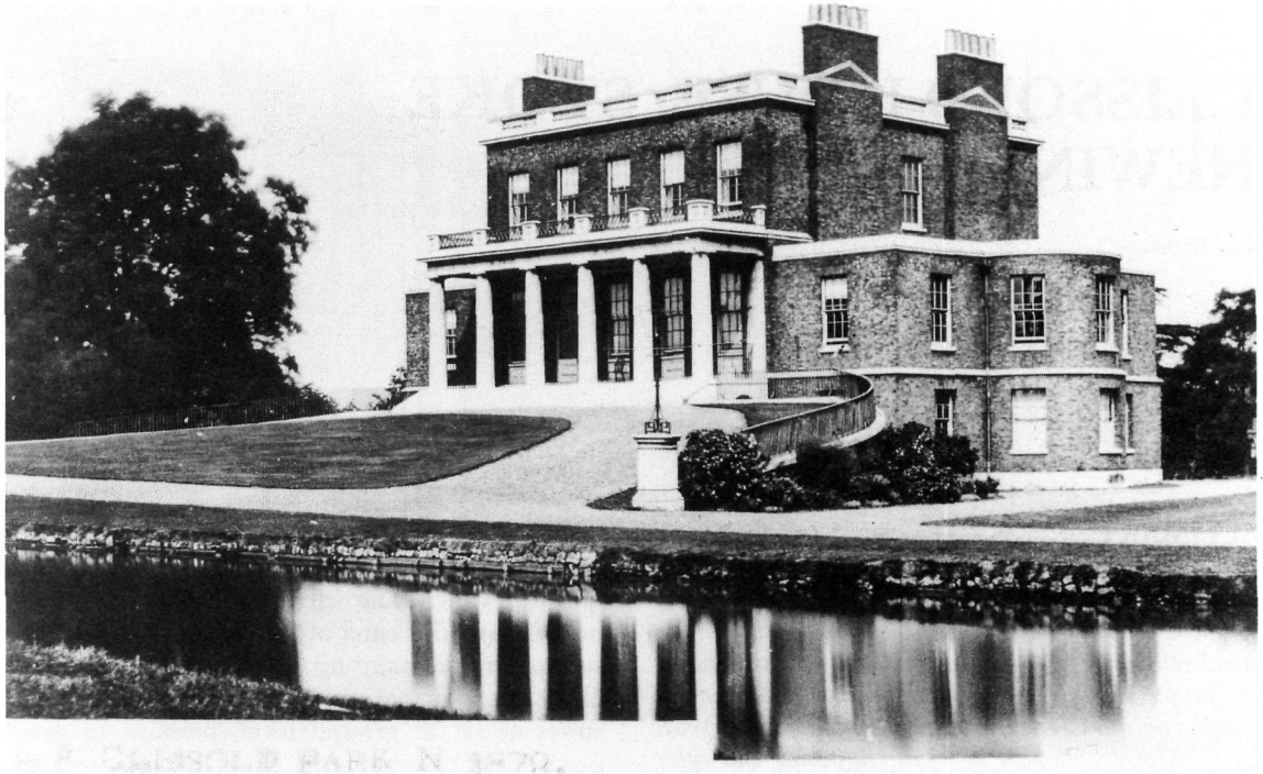
Fig 1. Clissold House from the south west, photographed in about 1876. The carriageway sweeps up to allow guests to enter the house on the middle floor level (courtesy Hackney Archives Department)
