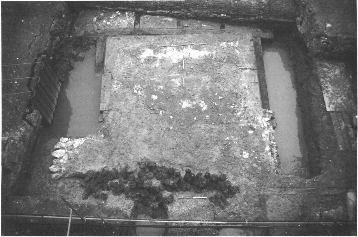
Fig 2. Trench 27 viewed from the parapet of the outer curtain wall in October 1996, towards the end of the excavation. In the foreground (east) is Feature 2954 and associated piling; a contemporary timber structure can be seen surrounding it and extending intact to the west. Some of the scattered timbers beyond were part of the framed structure – but others, unconverted beech trunks – may have been used in building work or incorporated in a temporary bridge. The massive round-backed feature crossing the trench is the culvert built during the backfilling of 1843–45 (Oxford Archaeological Unit)
