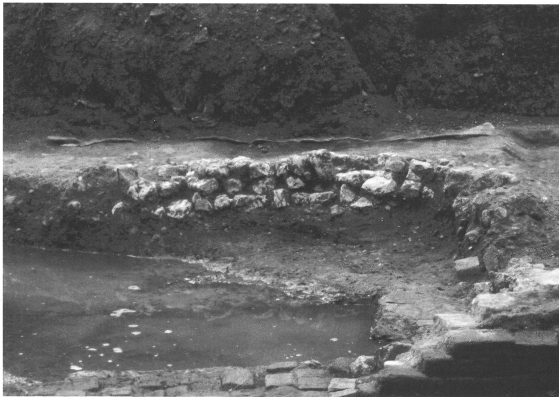
Fig 11. Structure 1 viewed from the north. The foundation measured 2.04m east-west
