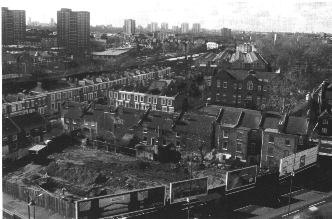
Fig 3. The excavations looking south-west
