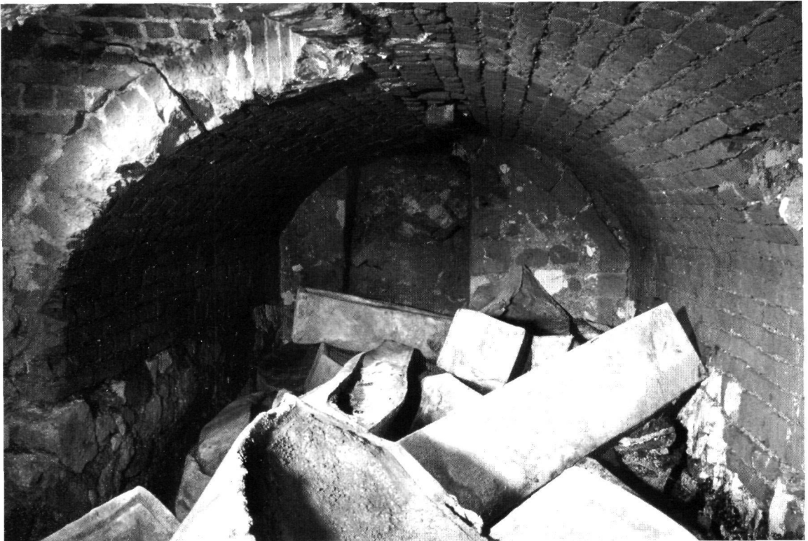
Fig 20. The vault looking north
