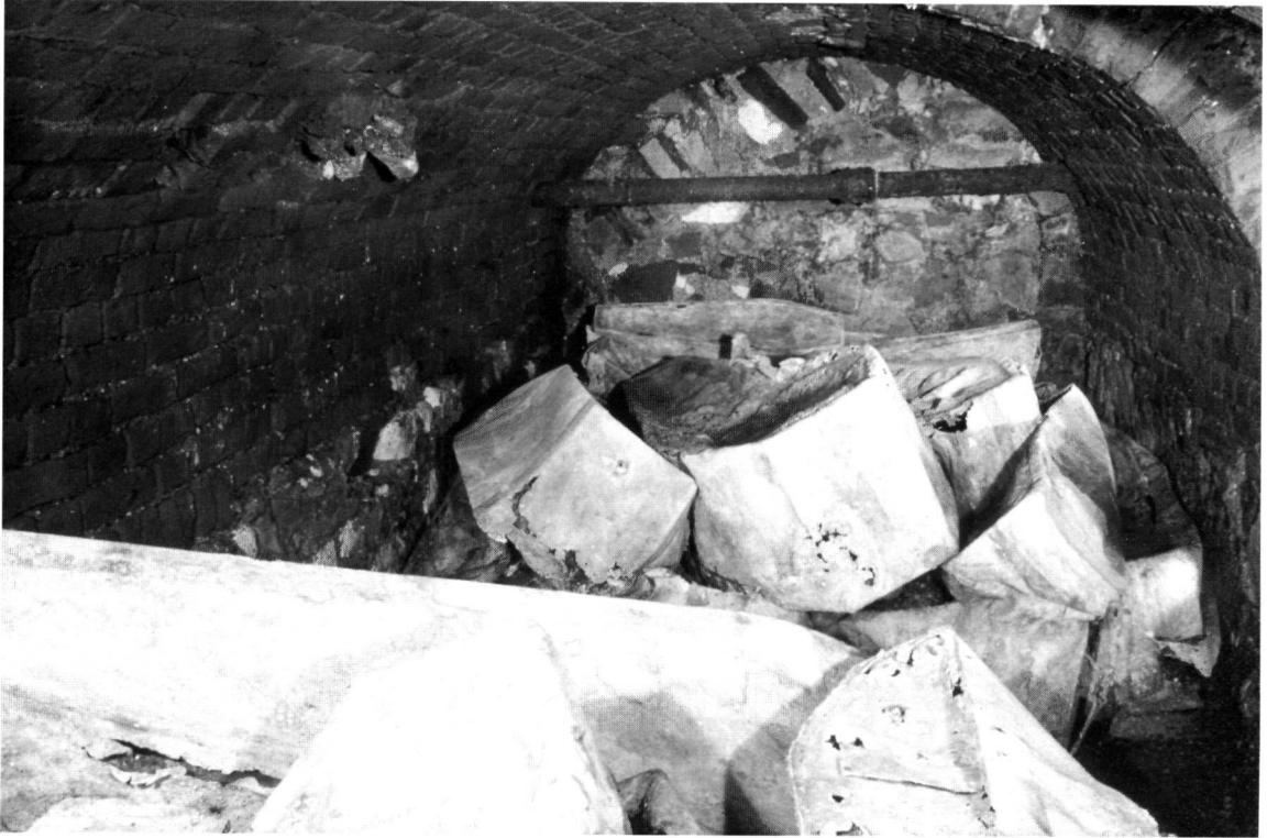
Fig 21. The vault looking south
